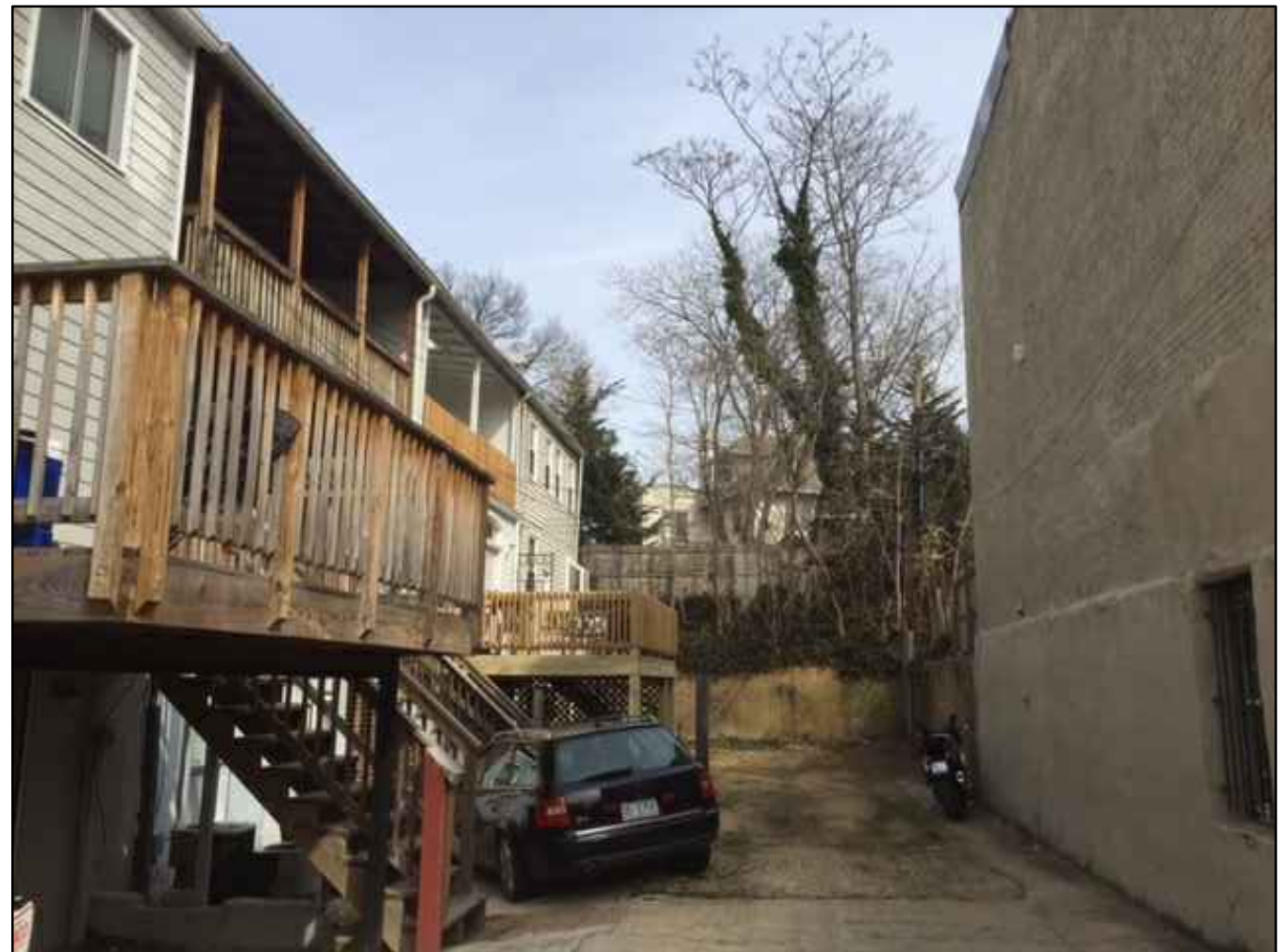
2 REAR VIEW LOOKING EAST C-5
