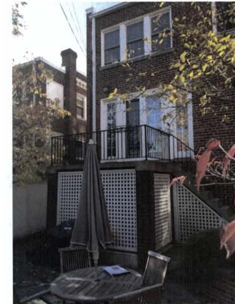
Existing View of Rear Deck and Stair
