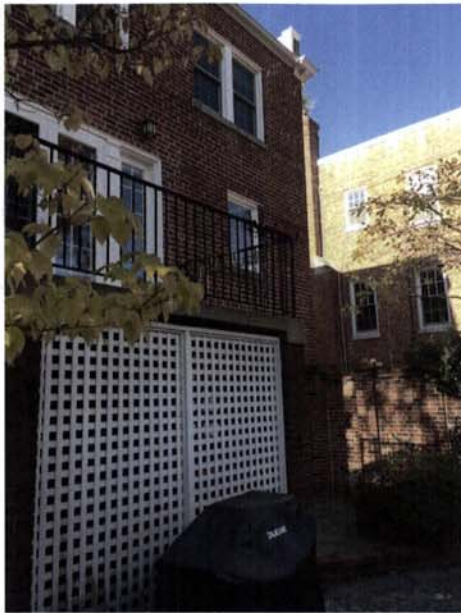
Existing View of Rear Deck and Stair
