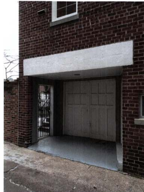
Existing View Garage
