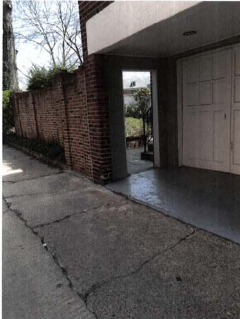
Existing View Garage/Rear Wall
