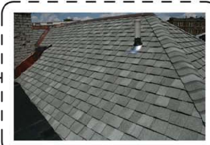
ASPHALT COMPOSITION SHINGLE ROOFING
