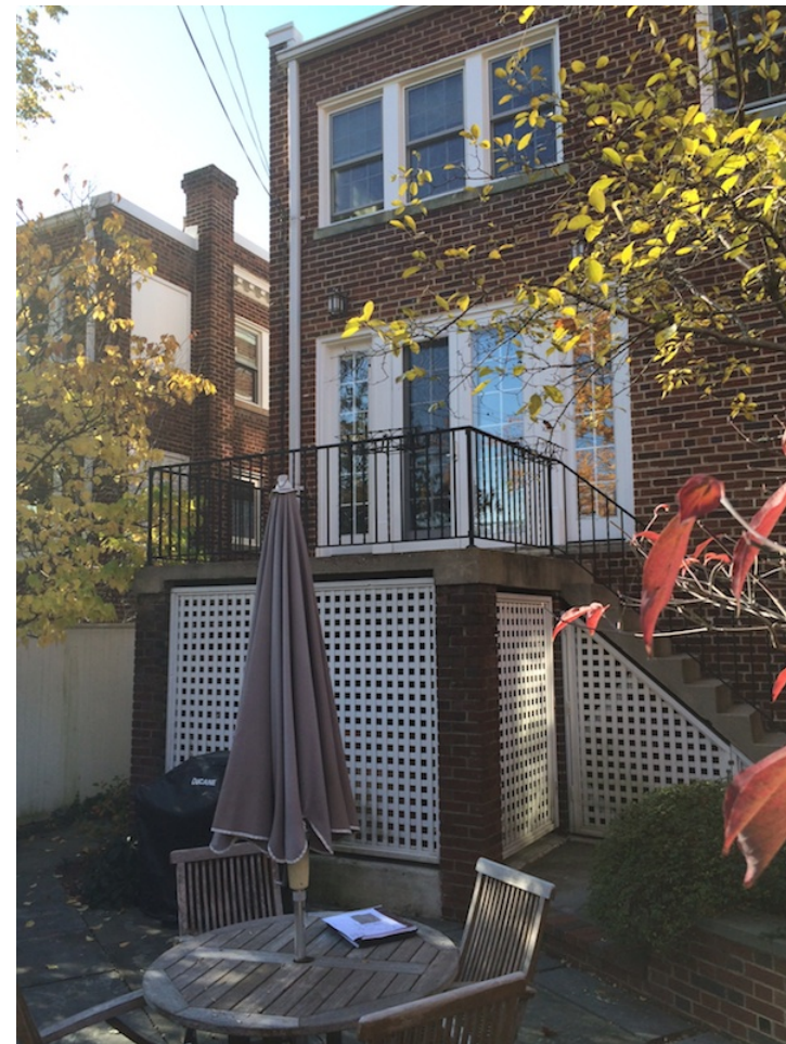
Existing View of Rear Deck and Stair
