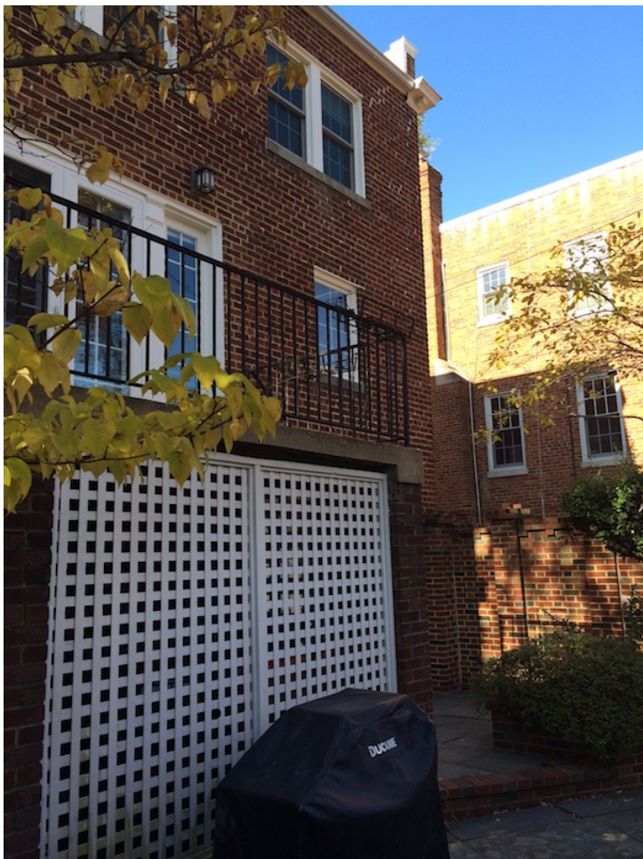
Existing View of Rear Deck and Stair
