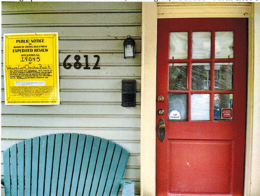
Photograph No. 2: 6812 Laurel St NW, Washington, DC 20012 – Porch Close Up
