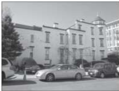
VIEW OF SITE/EXISTING BLDG. LOOKING SOUTHWEST; NOTE EXISTING CURB CUT.
