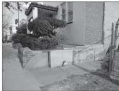
VIEW OF SOUTH EAST CORNER OF SITE/EXISTING BLDG. ALONG GEORGIA AVENUE.
