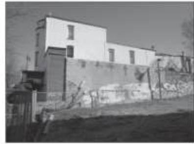
VIEW OF SITE/EXISTING BLDG. FROM GEORGIA AVE., LOOKING NORTHEAST
