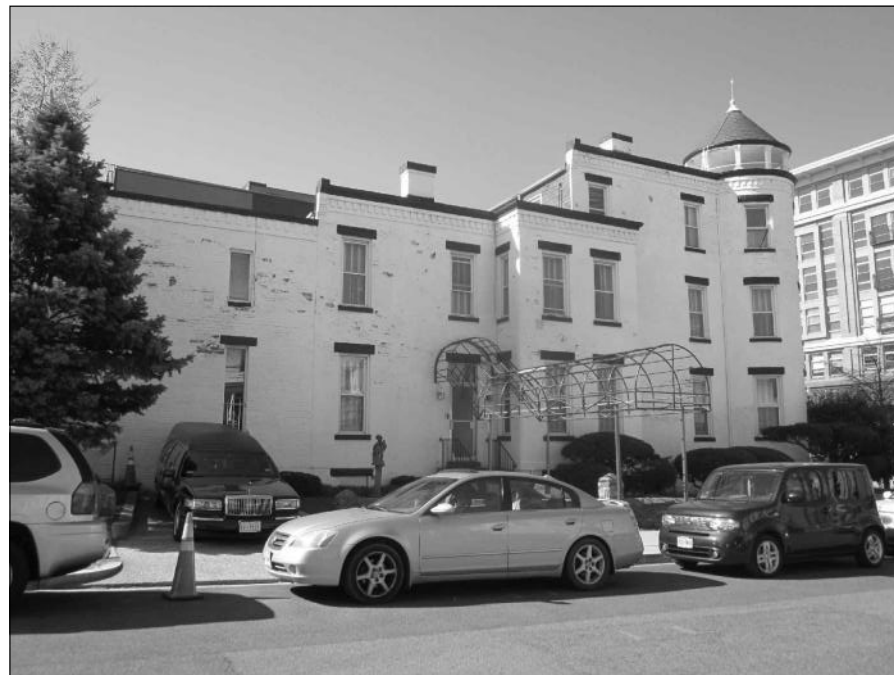
VIEW OF SITE/EXISTING BLDG. LOOKING SOUTHWEST; NOTE EXISTING CURB CUT.
