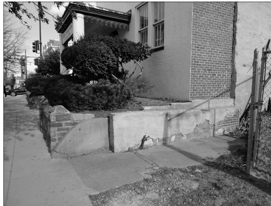
VIEW OF SOUTH EAST CORNER OF SITE/EXISTING BLDG. ALONG GEORGIA AVENUE.
