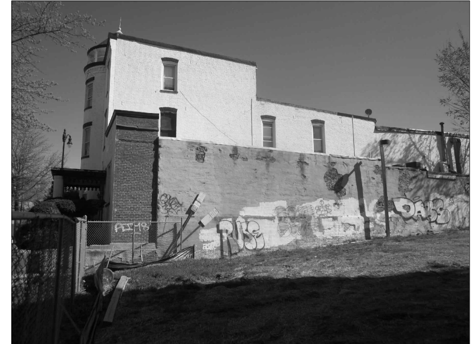
VIEW OF SITE/EXISTING BLDG. FROM GEORGIA AVE.; LOOKING NORTHEAST
