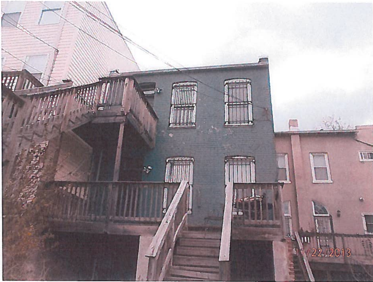
Previously existing deck situation at the subject property.
