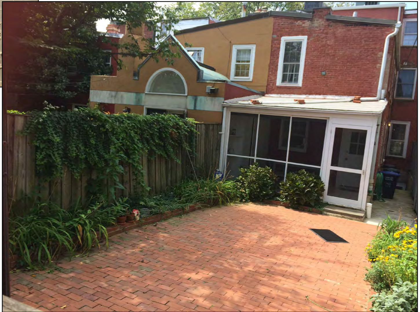
2 VIEW OF REAR, LOOKING SOUTH C-5
