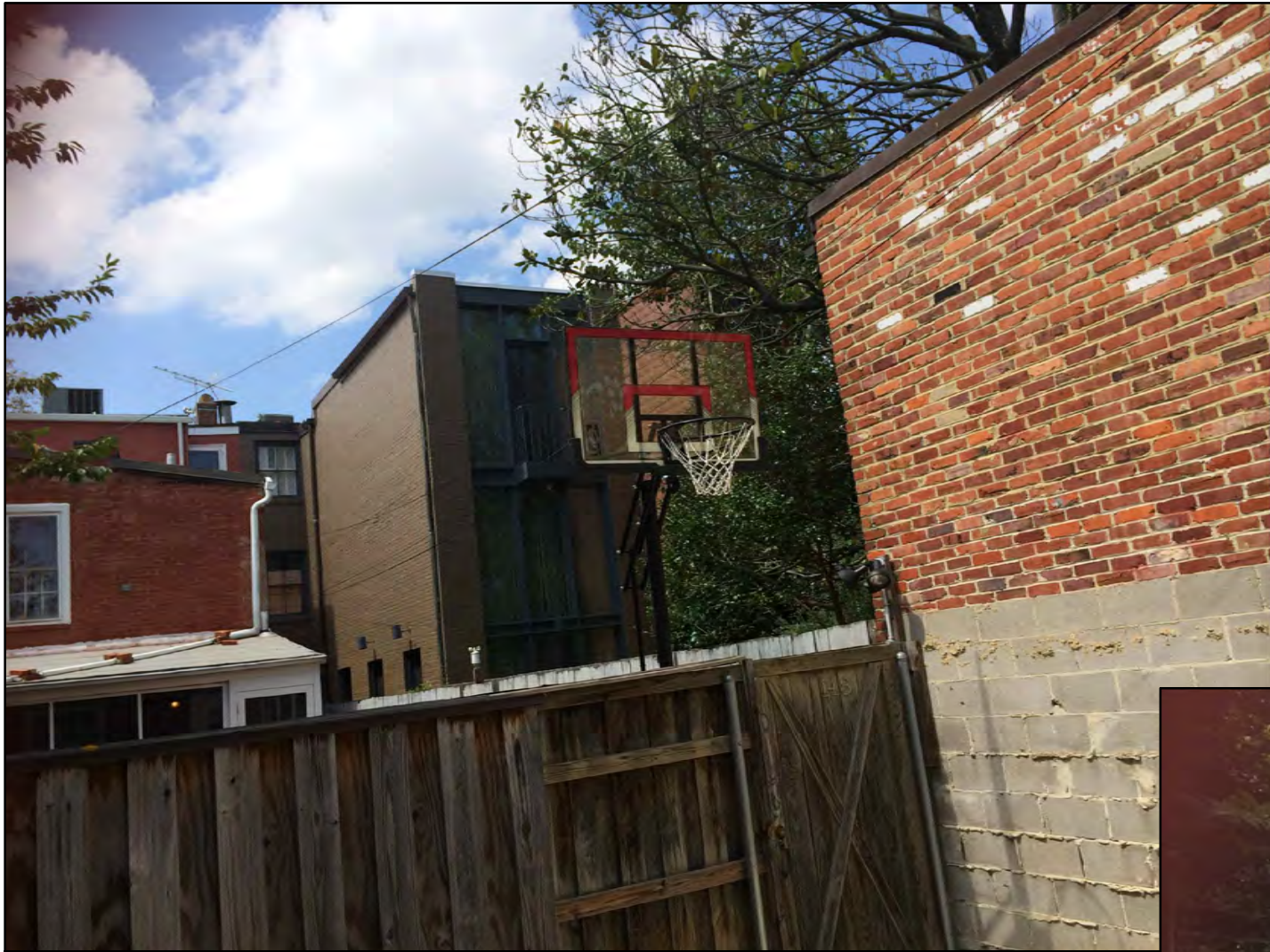
1 VIEW OF REAR, LOOKING NORTH C-5
