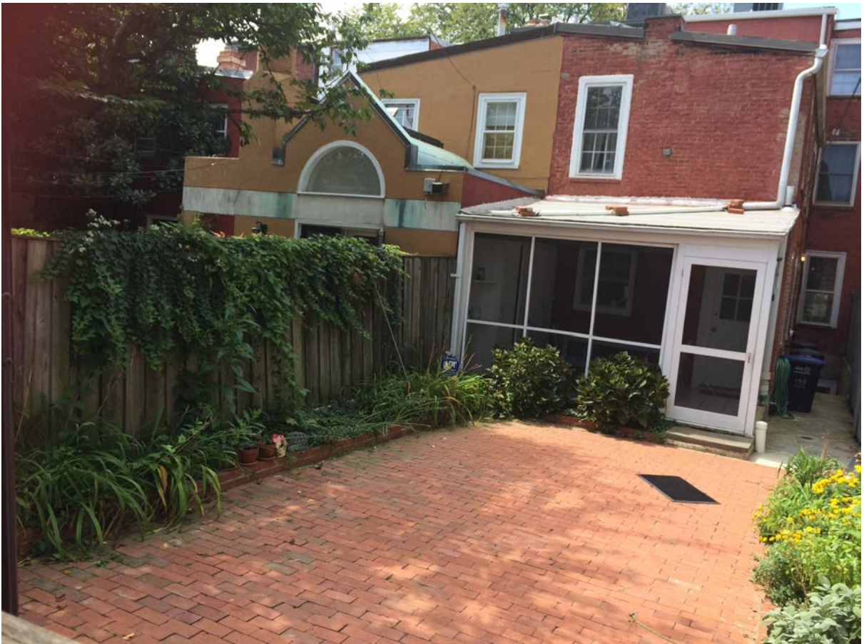
VIEW FROM YARD, LOOKING SOUTH
