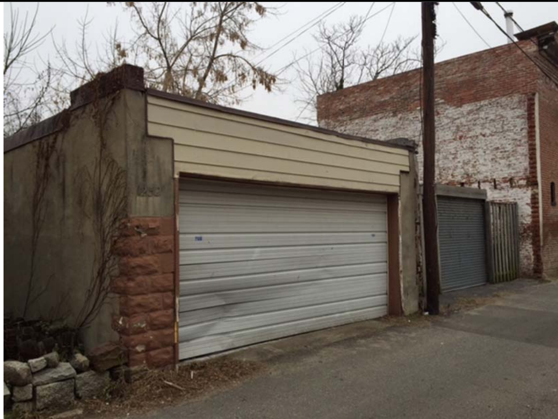
1 ALLEY VIEW, GARAGE @ 1252 FLORIDA AVE C-6 SCALE: NTS
