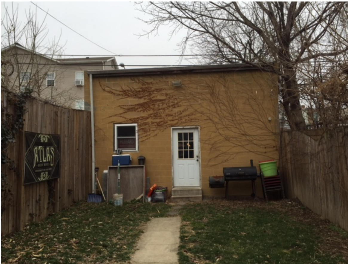
EXISTING GARAGE VIEW FROM YARD
