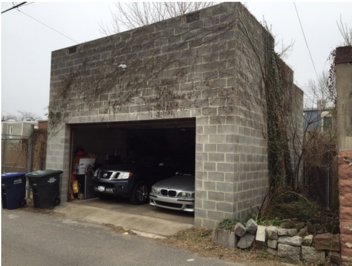
EXISTING GARAGE, VIEW FROM ALLEY
