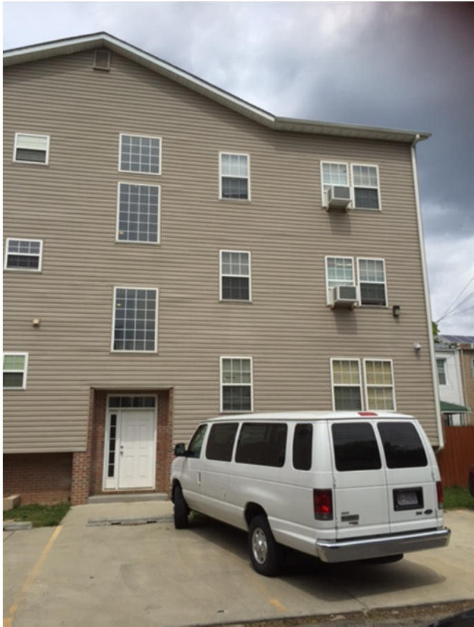
Three story structure across the alley from 1254 Florida Avenue NE
