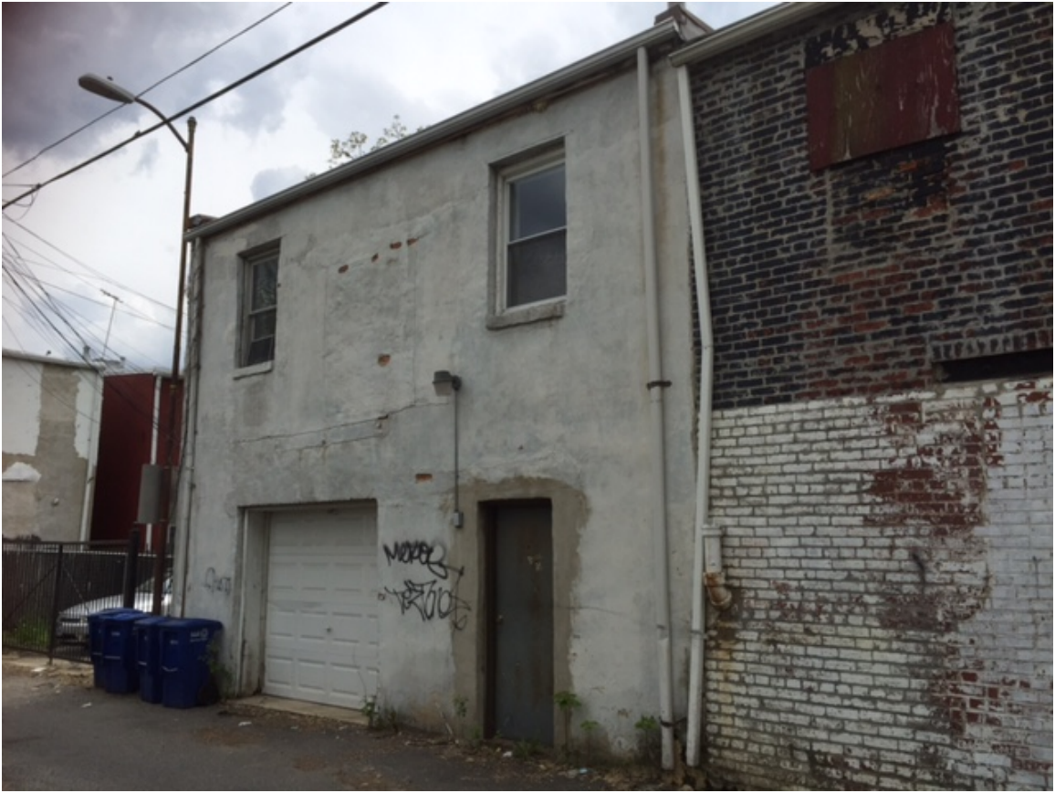
Example of a two story garage on the alley behind the 1200 block of Florida Avenue NE
