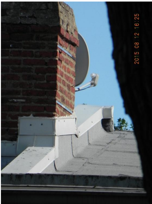
chimney detail 1519 Varnum
