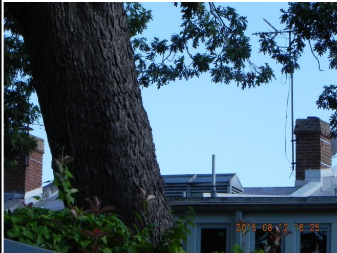
chimneys 1519 and 1521 Varnum
