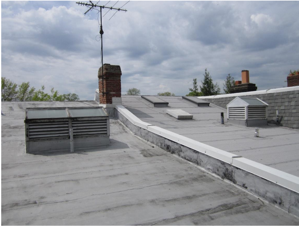
Photo No. 4: Roof Parapet between at 1521 Varnum Street, NW and 1519 Varnum Street, NW
