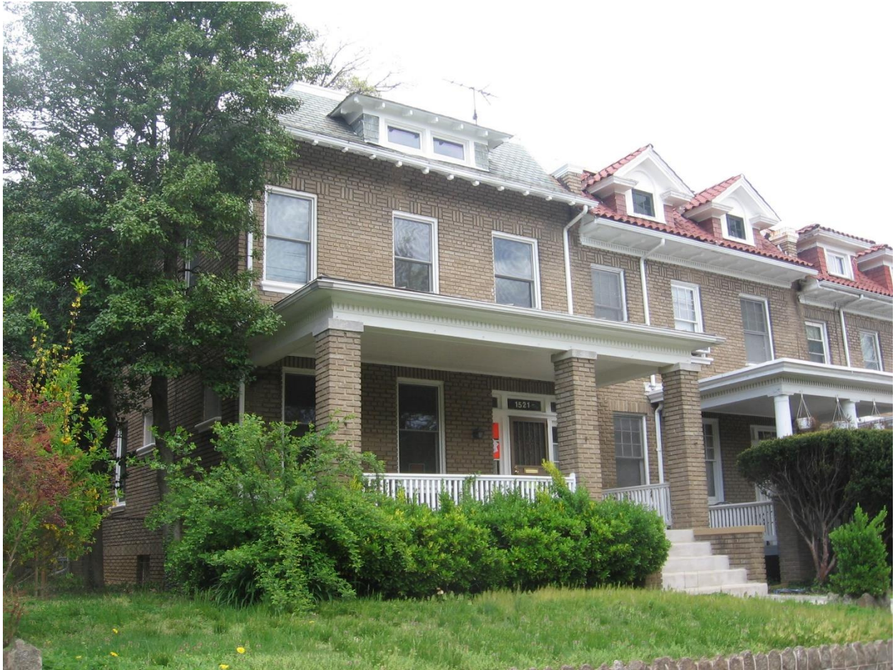
Photo No. 1: Front Elevation of 1521 Varnum Street, NW (Adjoining 1519 Varnum Street, NW property is to the right)
