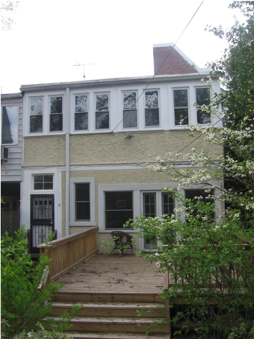
Photo No. 2: Rear Elevation of 1521 Varnum Street, NW (Adjoining 1519 Varnum Street, NW property is to the left)
