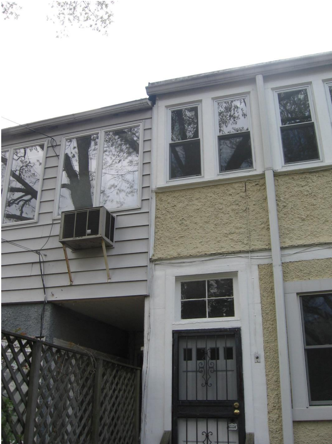
Photo No. 3: Party Wall at Rear Elevation (Between at 1521 Varnum Street, NW and 1519 Varnum Street, NW)
