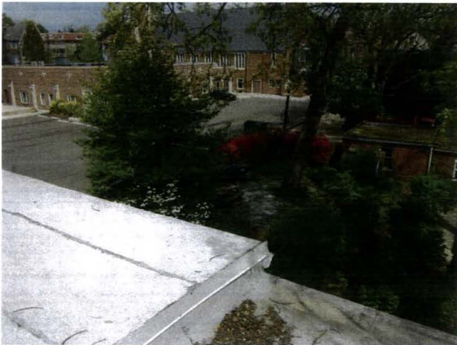
Photo No. 5: Roof Parapet between at 1521 Varnum Street, NW and 1519 Varnum Street, NW
