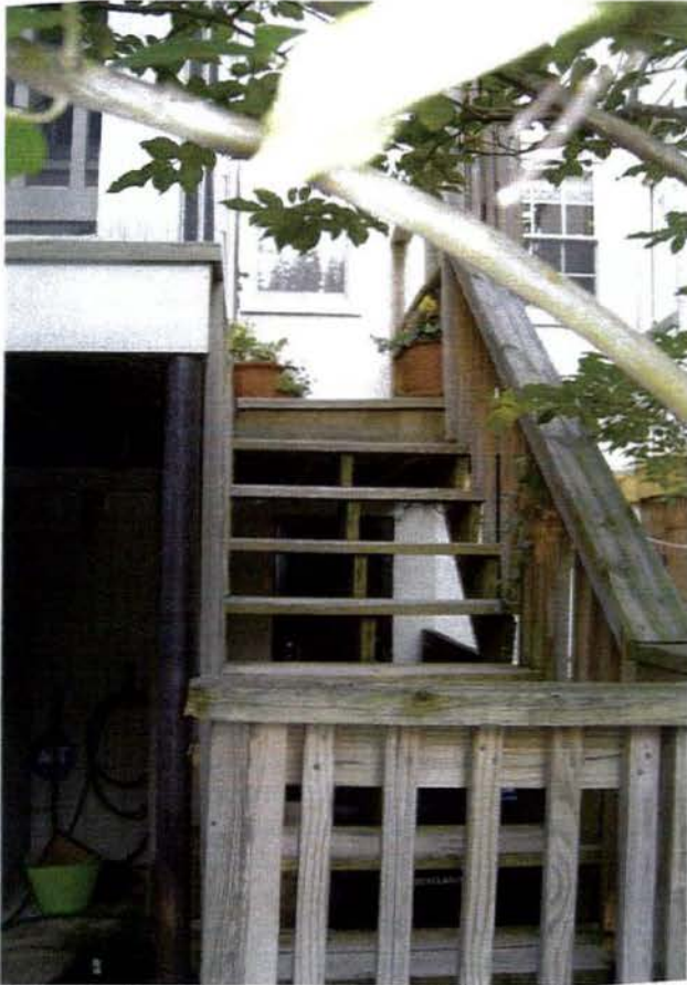
Stairs to landing – porch on left, applicants' property to right
