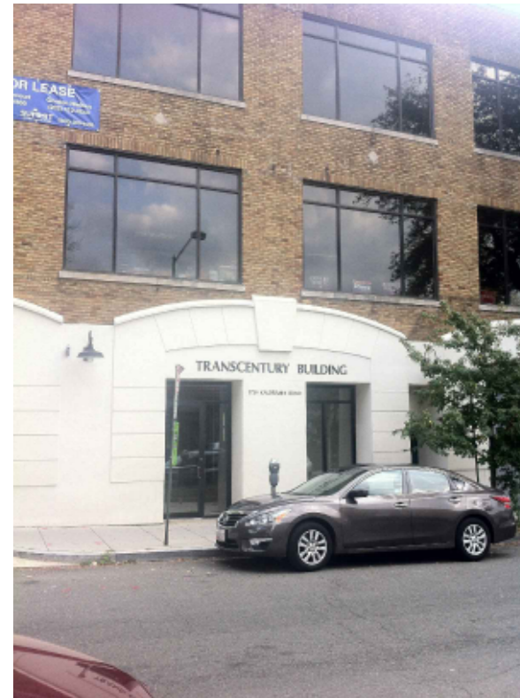
EXISTING FRONT ENTRY
