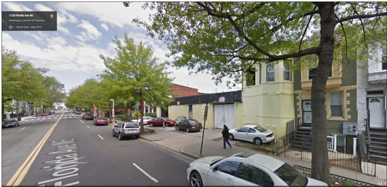
FRONT OF STRUCTURE FROM FLORIDA AVENUE LOOKING NORTHWEST
