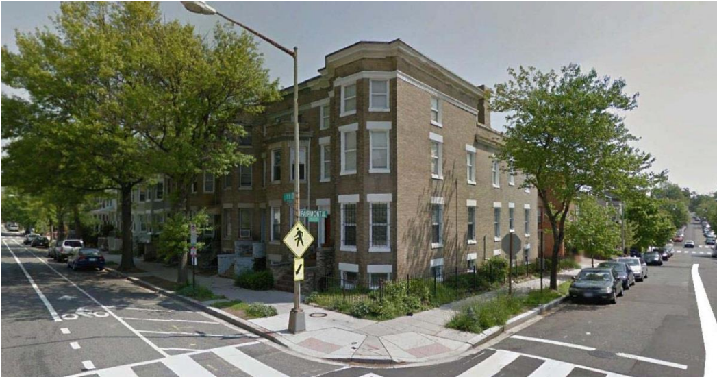
Fig. 2. Shows the large amount of fenestration provided by the corner property.
