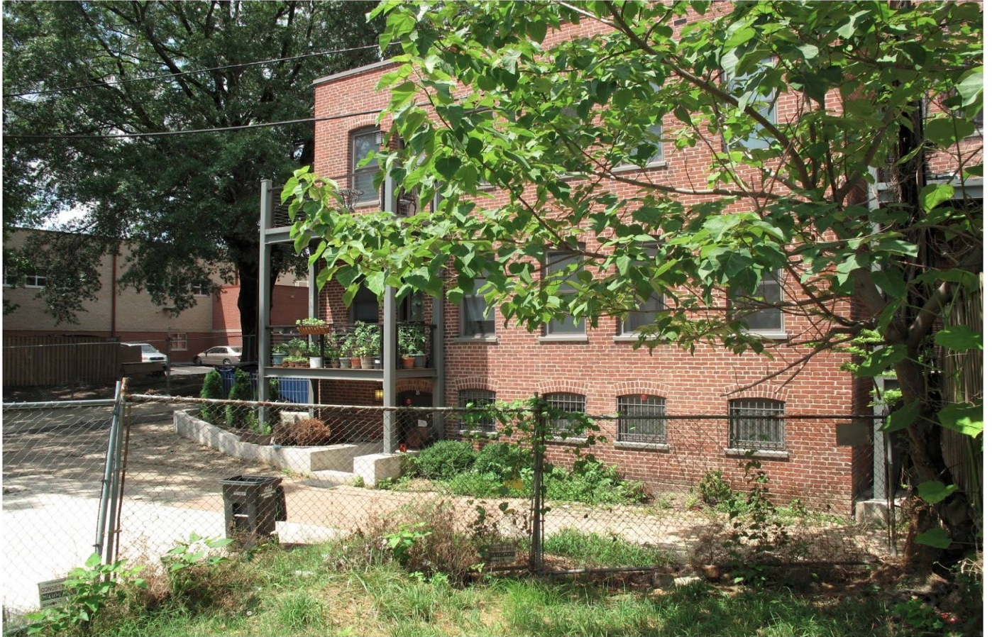
New construction immediately across alley housing eight units. Photo shot from rear yard of the Applicant's property.
