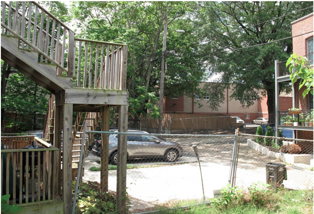
Immediate neighbor's wooden deck extending this property's lot occupancy beyond 70%.
