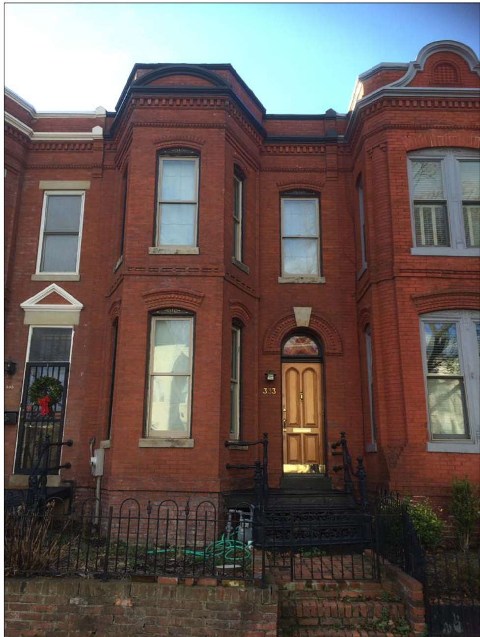
Street Frontage 333 F Street NE
