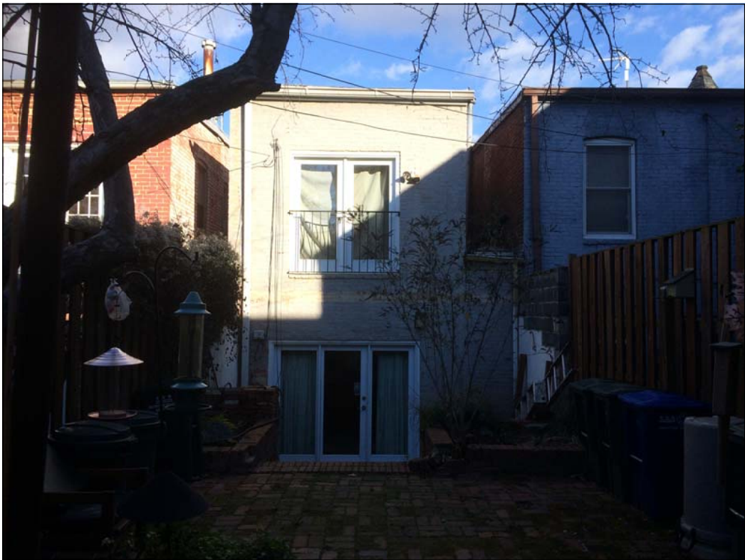
View of 333 F Street NE from Rear Yard
