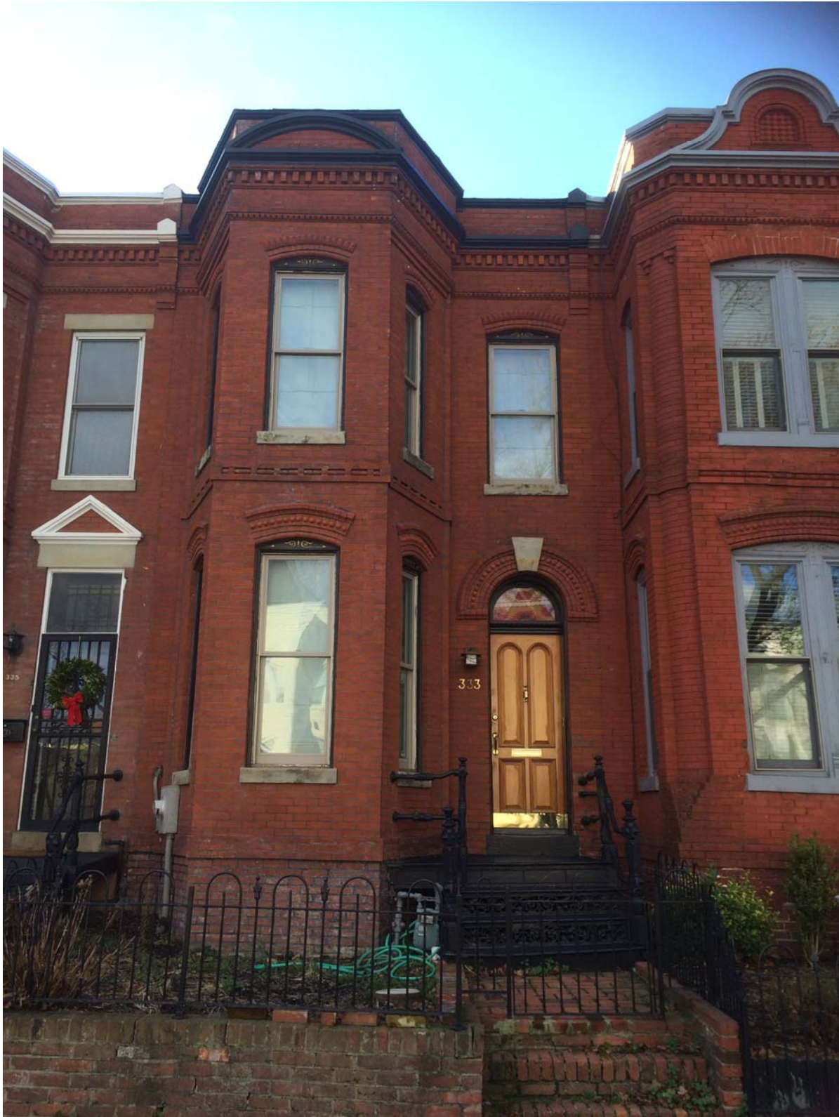
Street frontage of 333 F Street NE
