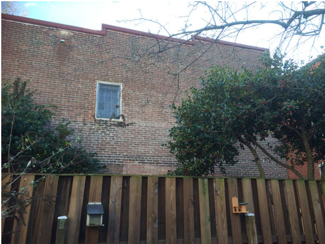
View East from rear yard
