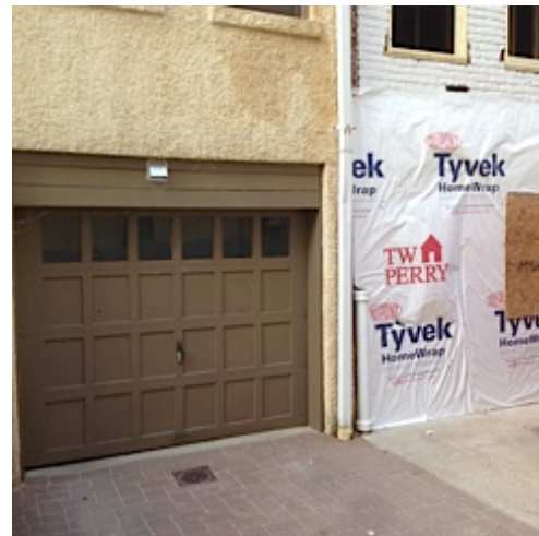
Rear West Perimeter (with garage Door down)
