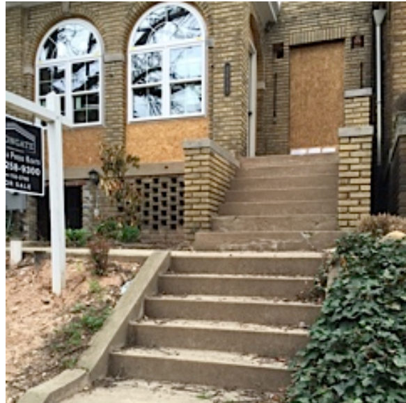
Stairs to First Landing
