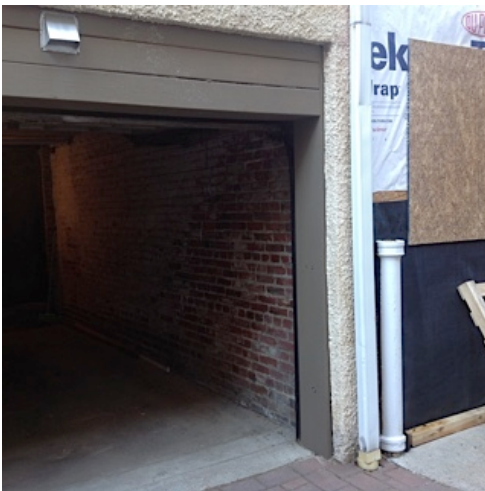
Rear West Perimeter (with garage Door up, accessible for measurement)
