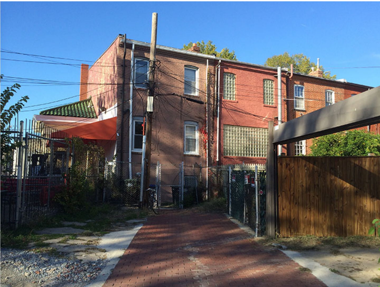
EXISTING REAR VIEW OF BUILDING SHOWING NEIGHBORS
