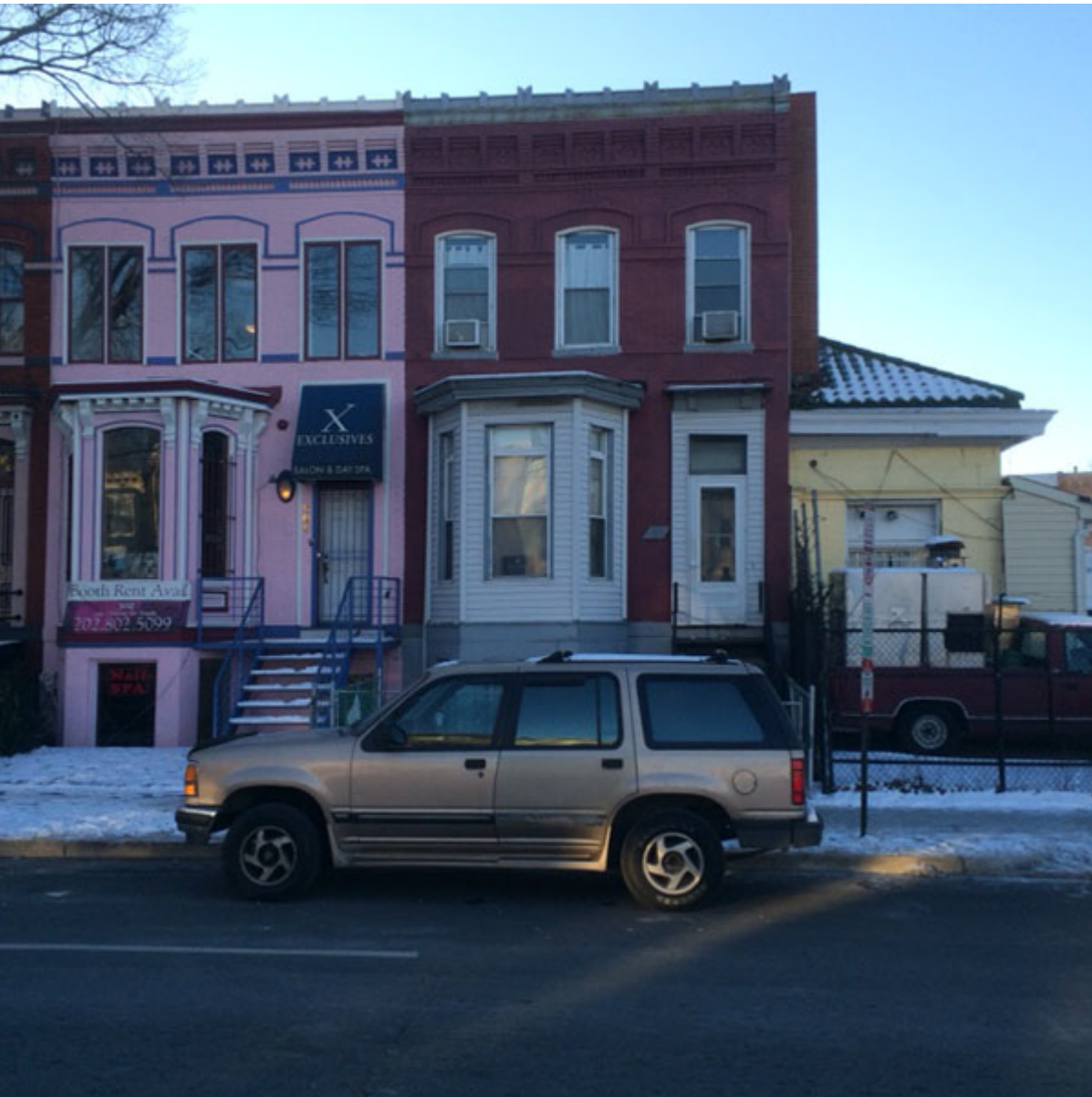
EXISTING FRONT VIEW OF BUILDING SHOWING NEIGHBORS TO THE WEST
