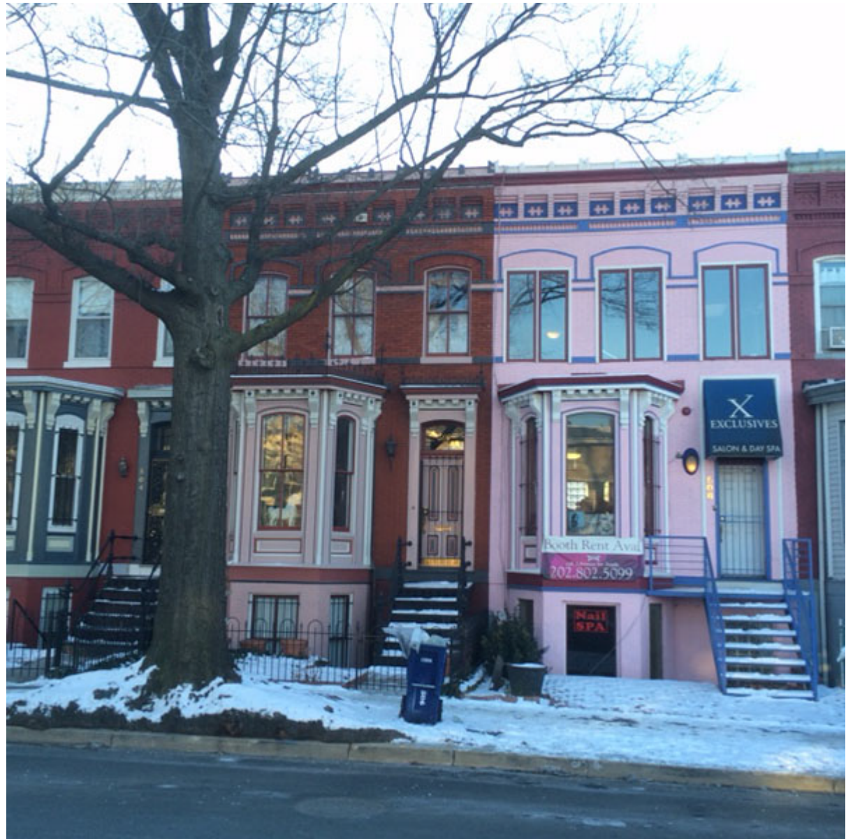
EXISTING FRONT VIEW OF BUILDING SHOWING NEIGHBORS TO THE EAST
