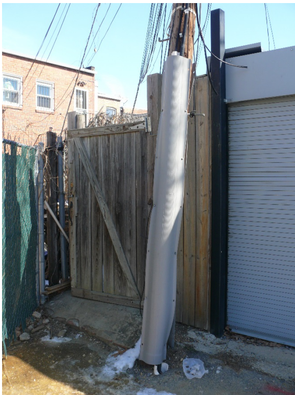
Gate to private walkway across rear of 413 H St NE
