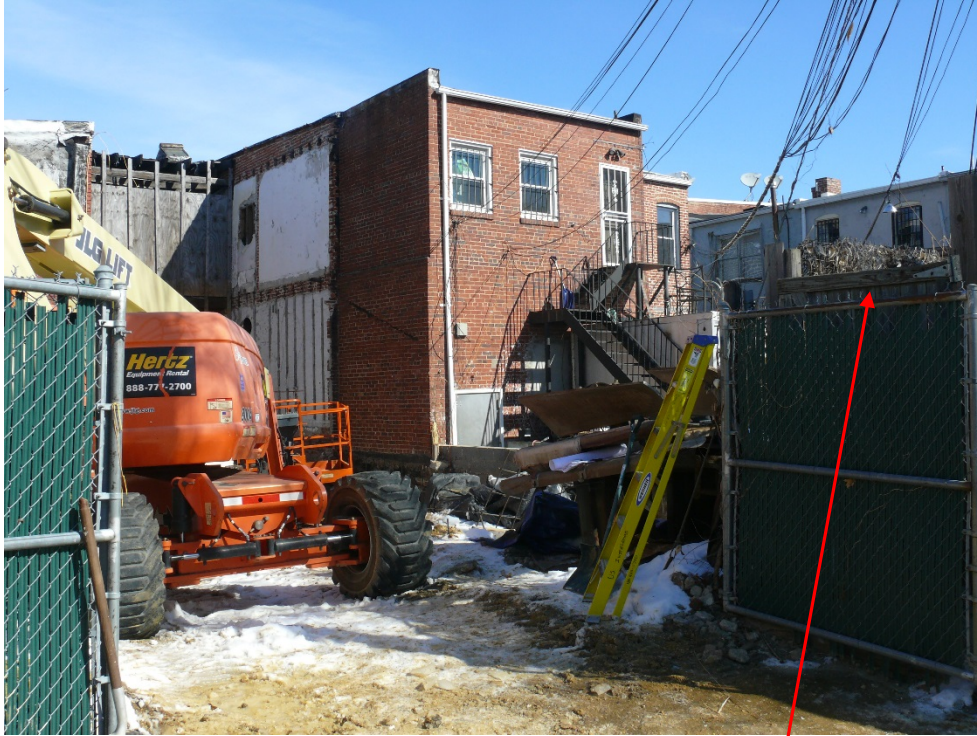
Rear 411-13 H Street, N.E. Private walkway located behind construction gate to right in photograph
