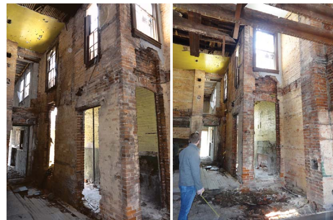
Photos of existing brick walls in existing space -- Walls to remain and openings to be adjusted in order to retain the existing character of this structure and allow stair to interact with it
