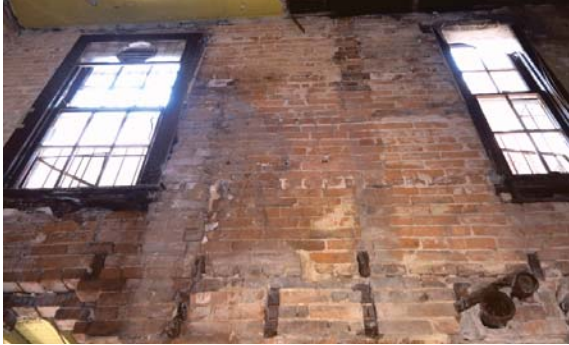
Maintaining character of existing building elements and brick for "patchwork walls."
