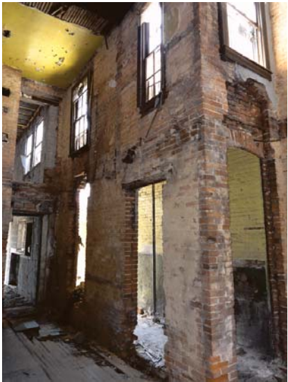
Photos of existing brick walls in existing space
