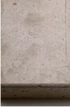
Light concrete countertops at Bev/Cond cabinet
