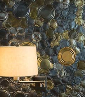
Painted can tops at wall surface in niche
