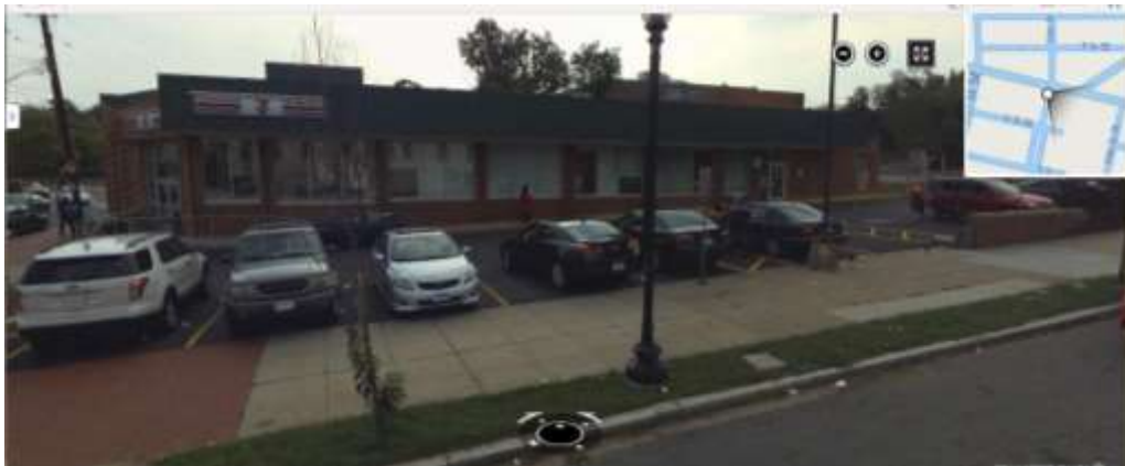
Front of Building along 14 th Street
