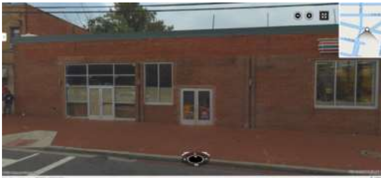
Front of Restaurant along Good Hope Road
