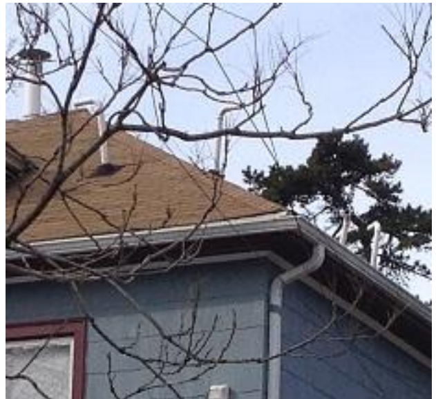
North side – four vents
