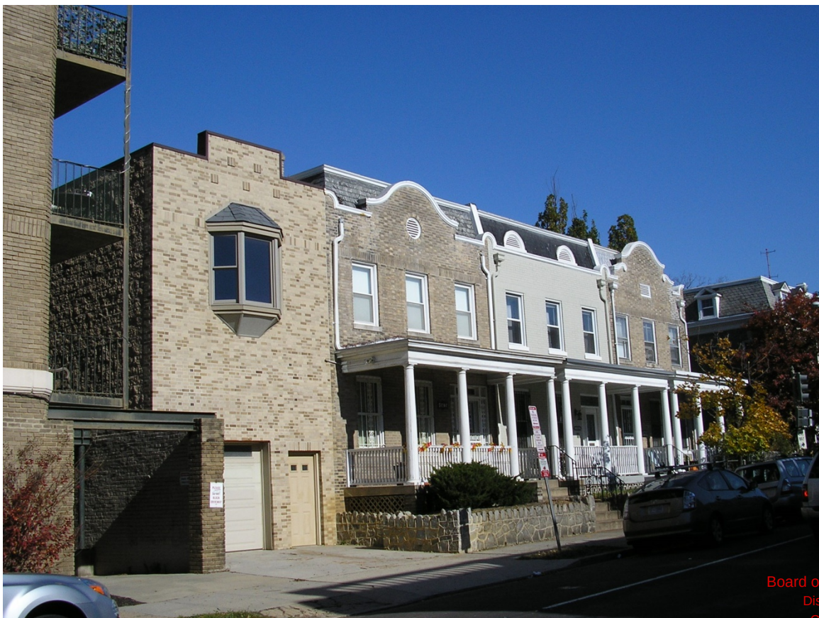
Bottom: 1505 Harvard Street with addition on left. Note mansard roof behind a parapet wall.
