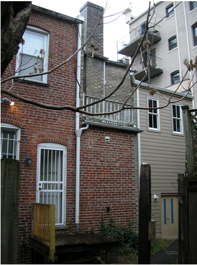
1505 Harvard Street rear yard looking to the southwest.
