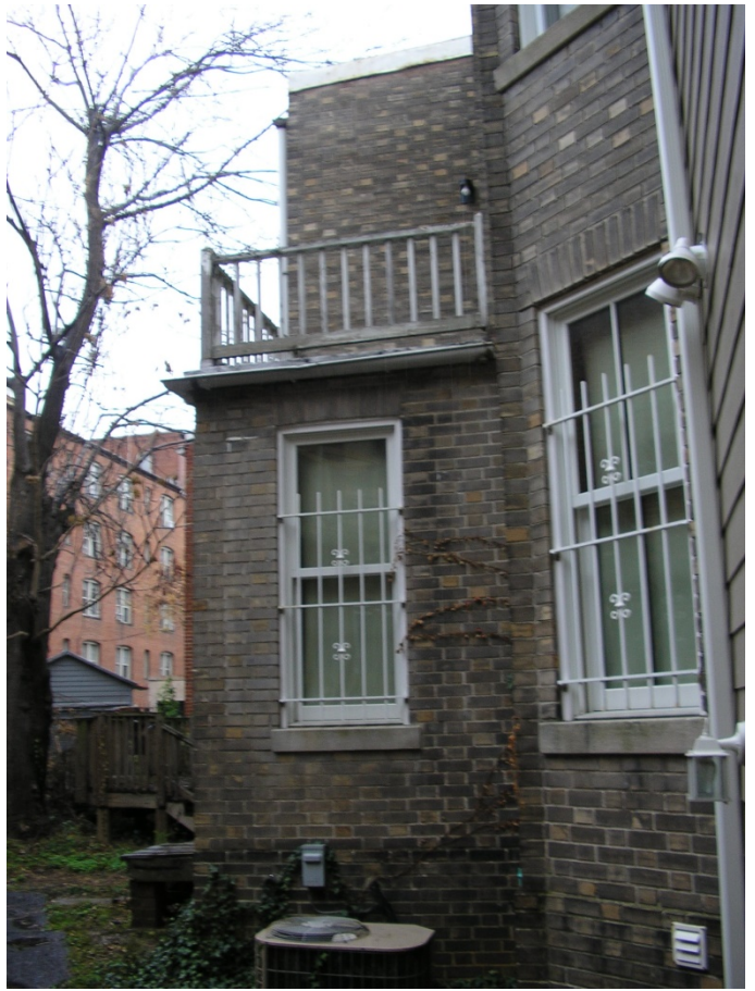
Rear yard looking to the northeast. Note second floor walk-out porch that will be converted to a walk-in closet, this will add to rear neighbors' privacy.
