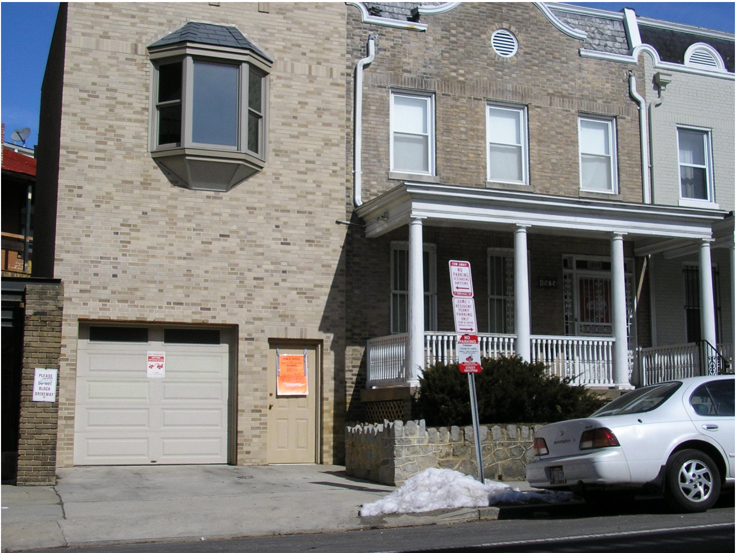
Photograph No.1 Harvard Street Frontage – Across From 1505 Harvard Street
