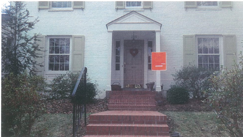
Photograph 2. Posted on building. Street frontage 3318 Fessenden St NW, Washington, DC 20008.
