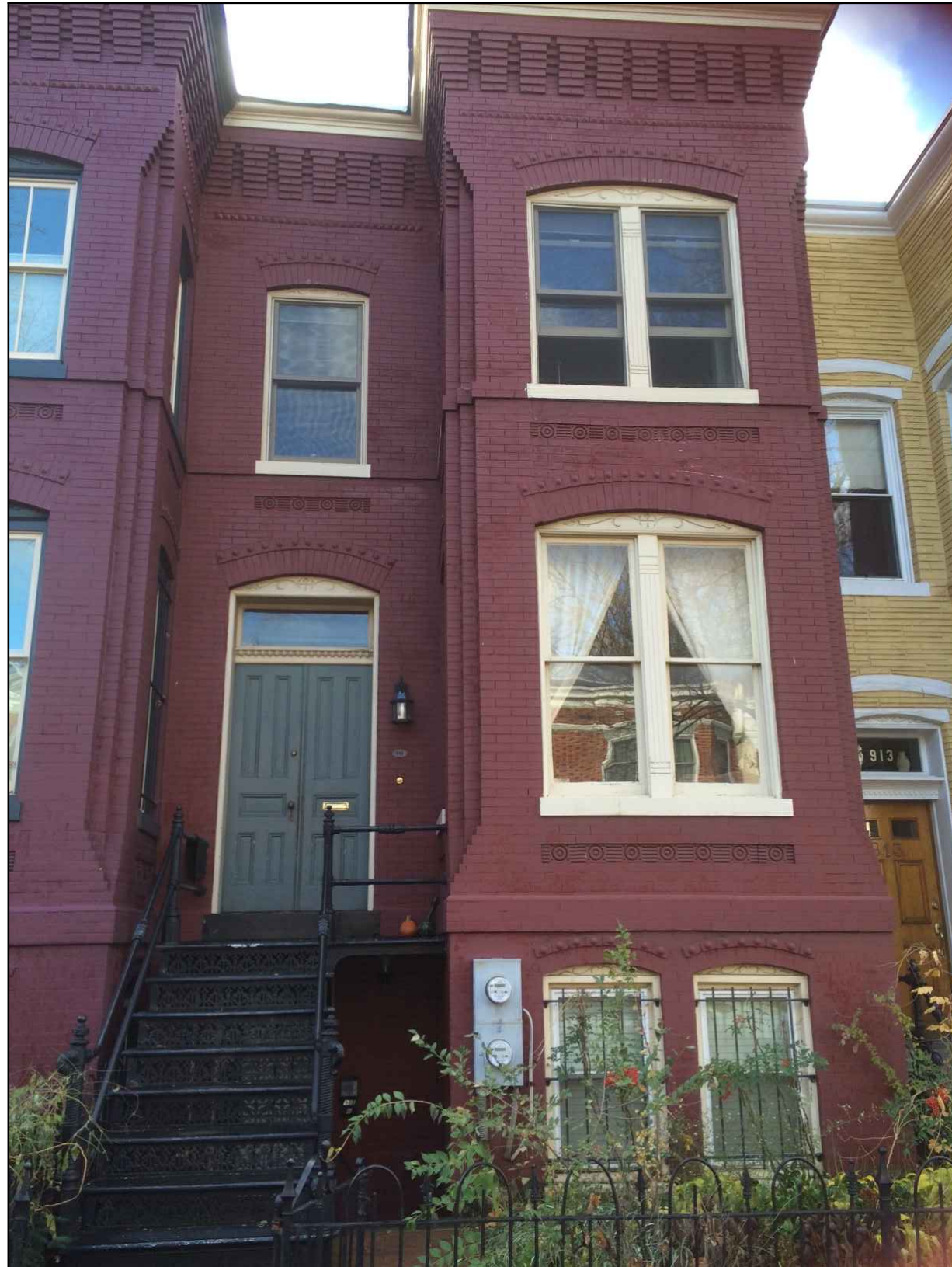
1 FRONT OF HOUSE, 915 C STREET NE C-4
