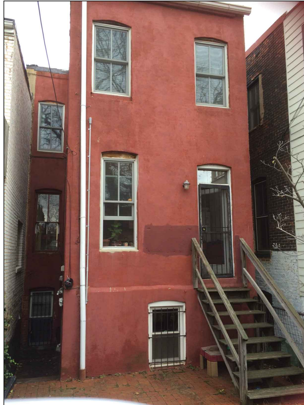
2 REAR OF HOUSE, 915 C STREET NE C-4
