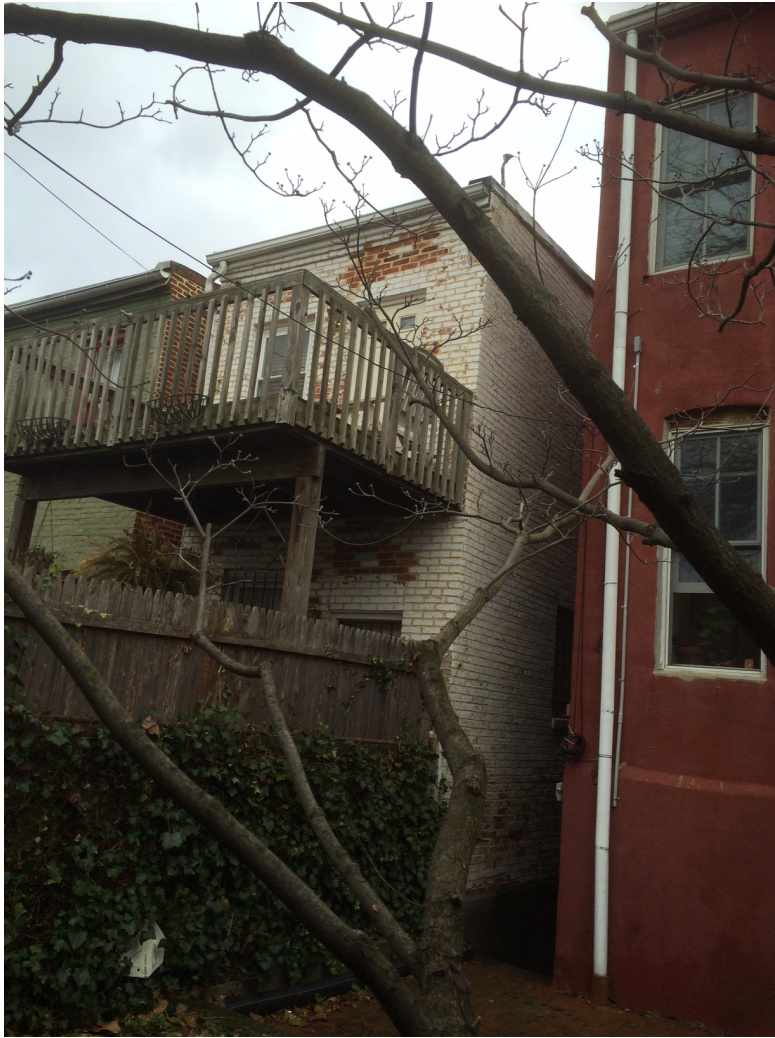
VIEW TO WEST OF 915 C STREET NE
