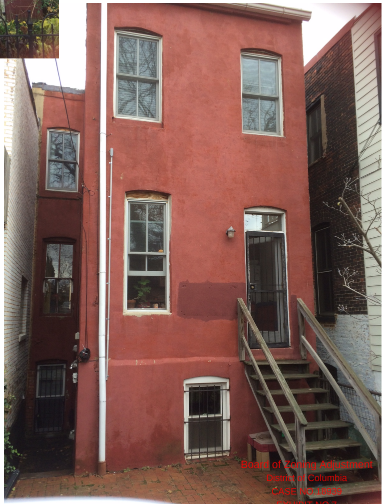
REAR OF HOUSE, 915 C STREET NE
