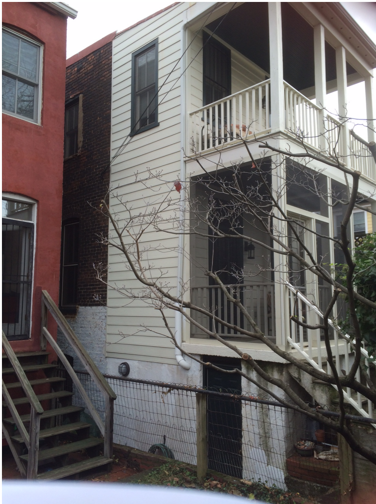
NEIGHBOR TO EAST OF 915 C STREET NE
