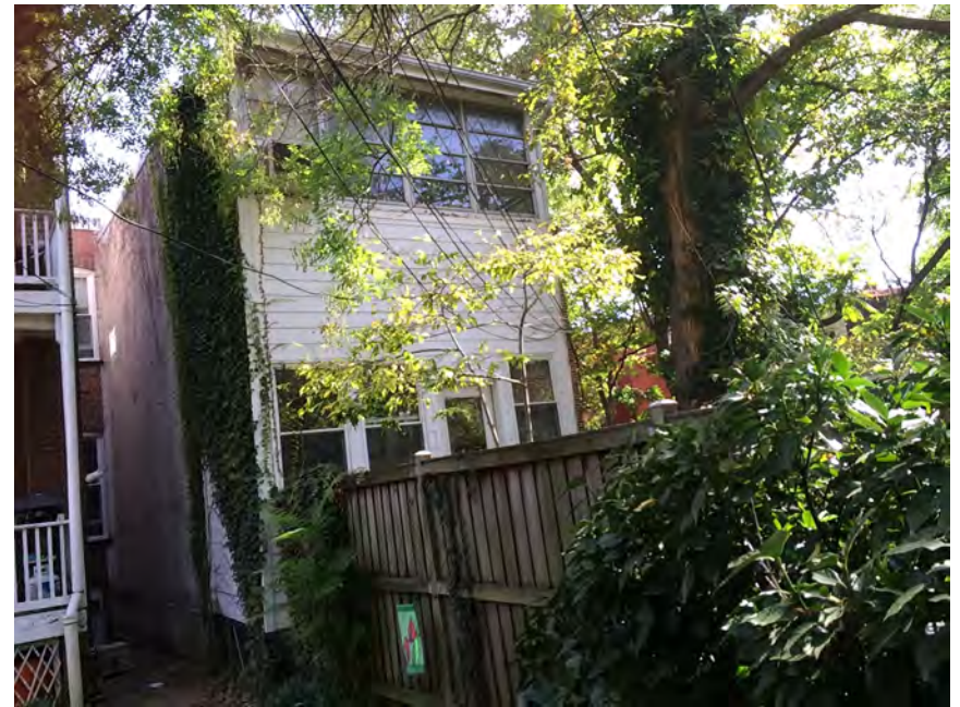
REAR YARD, LOOKING SOUTH
