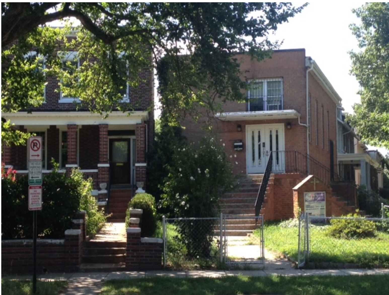
1401 South Carolina Avenue SE: SC Ave façade
