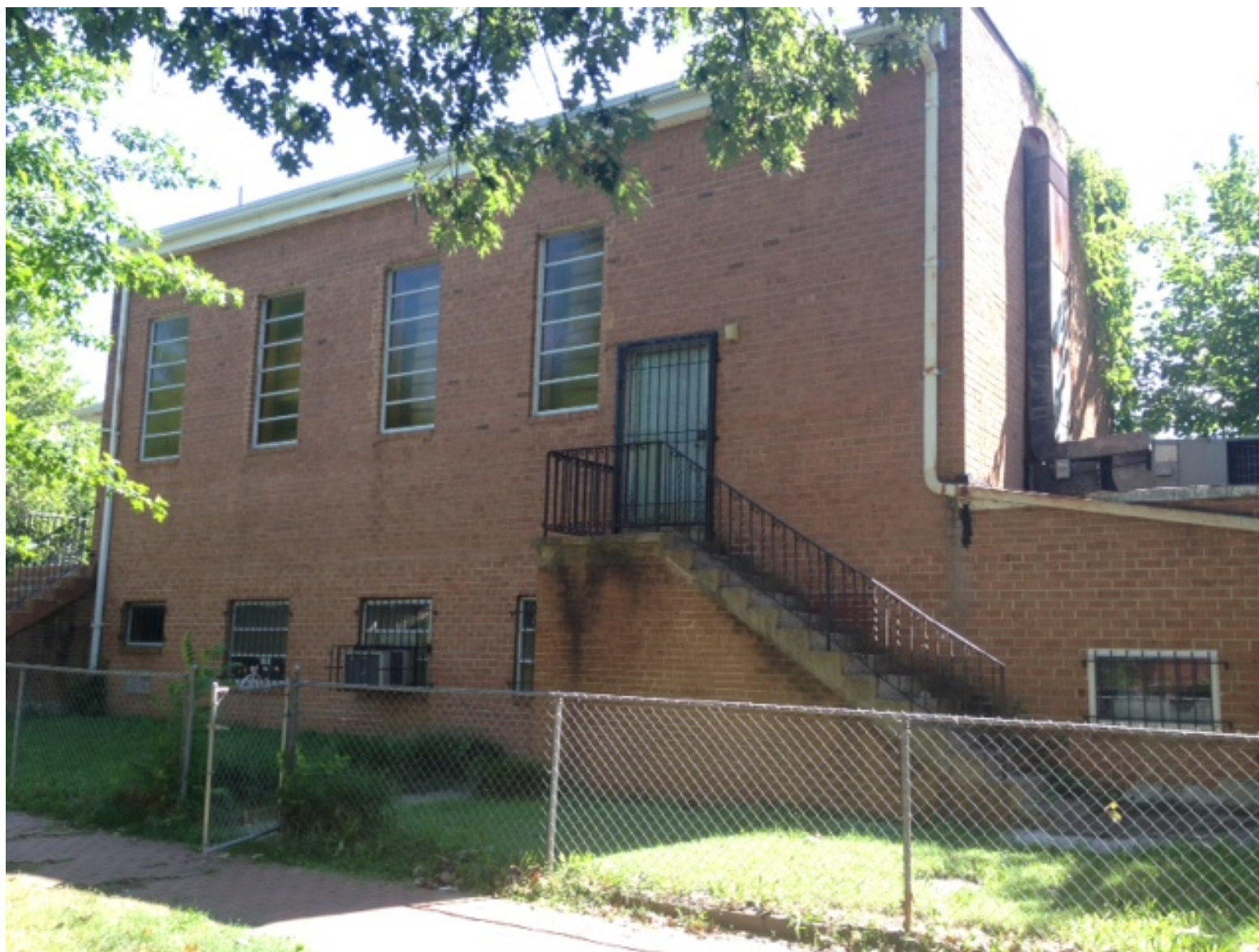
1401 South Carolina Avenue SE: 14 th Street façade
