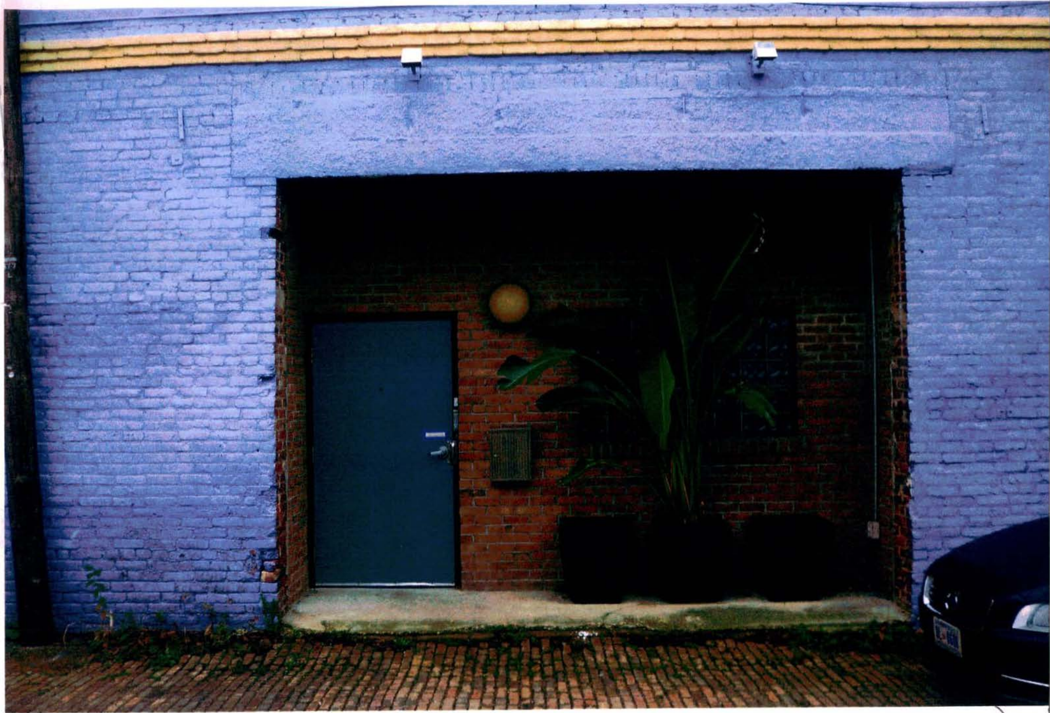
#37 LOT 81 PARTIAL VIEW, NORTH (MID-WEST)
