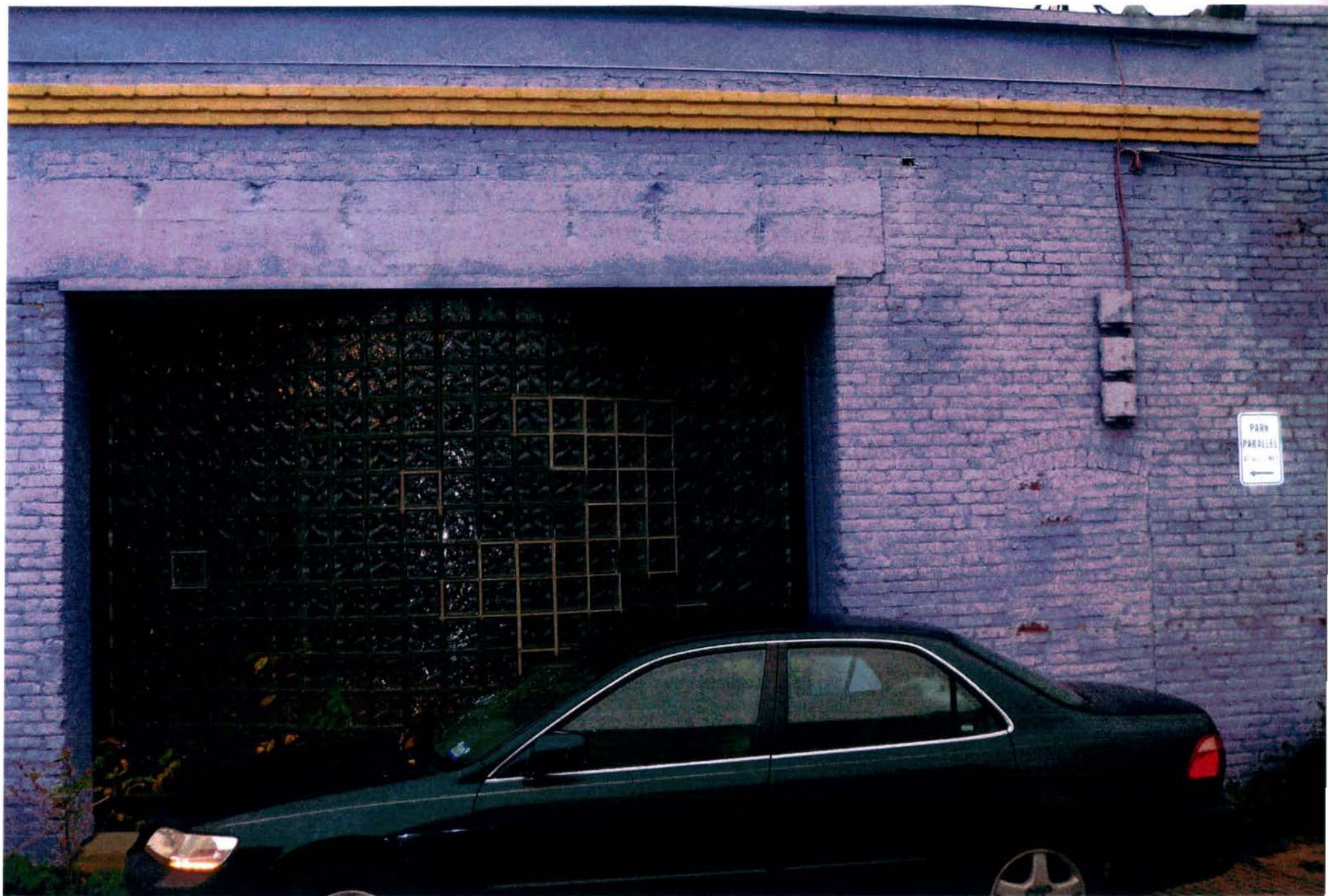
LOT 81 PARTIAL NORTH VIEW (MOST WEST) #36
