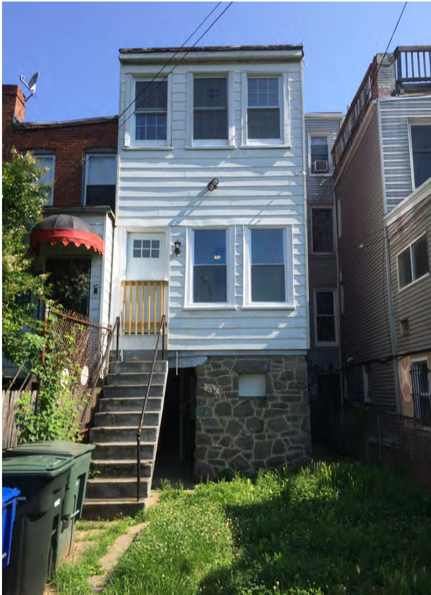
REAR FACADE, 34 V STREET NW
