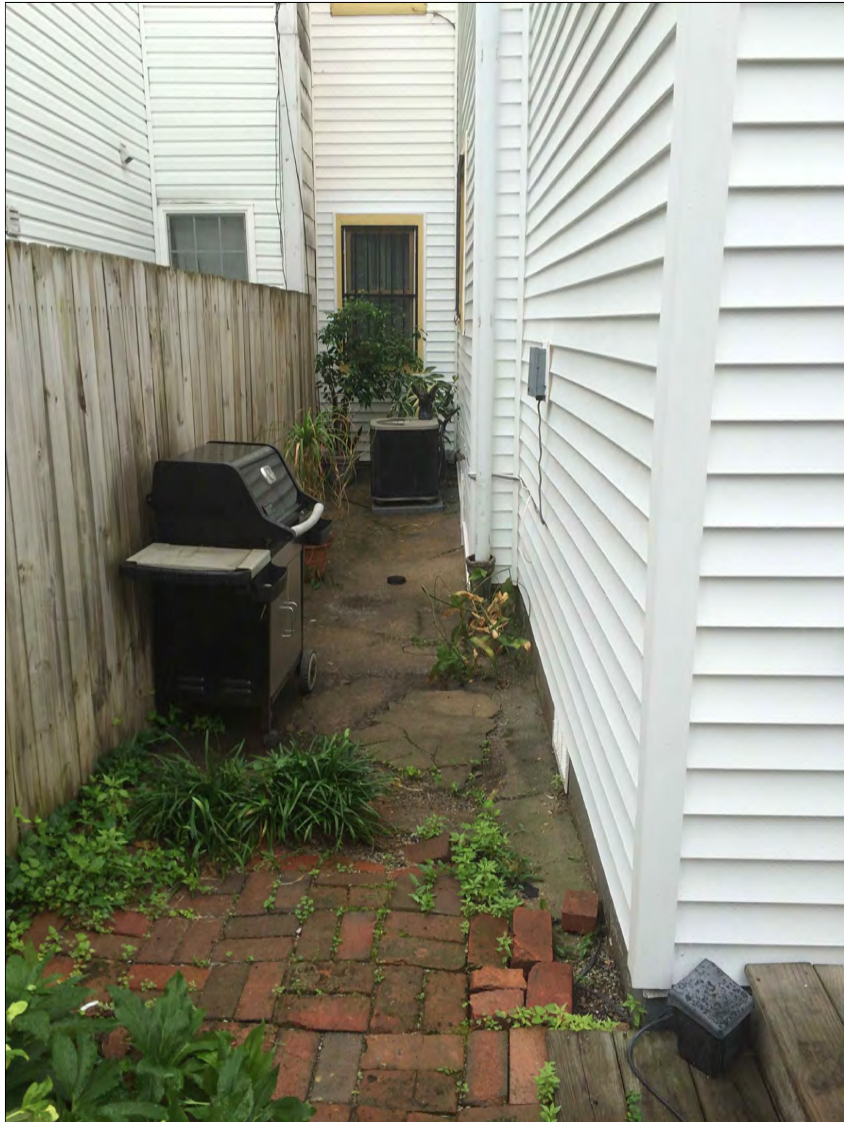
2 C-6 VIEW OF DOGLEG FROM YARD
