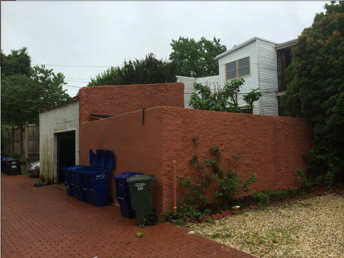
2 C-4 EXISTING GARAGE, LOOKING EAST
