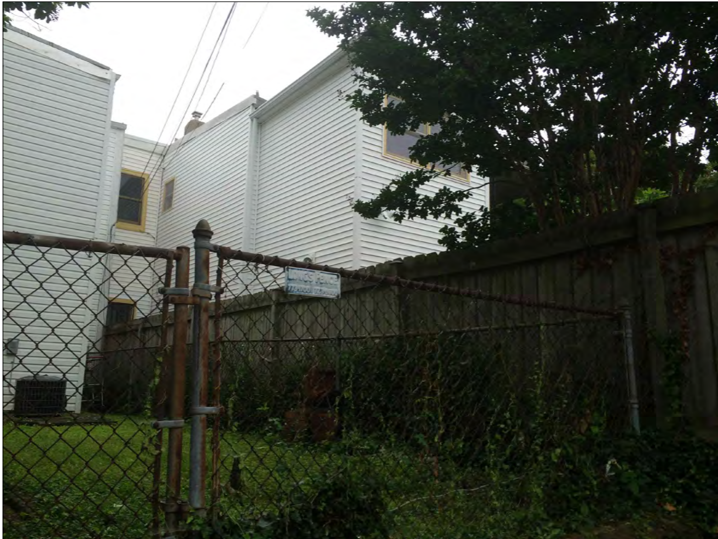
1 C-6 VIEW OF DOGLEG FROM ALLEY
