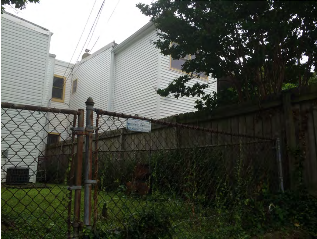
VIEW OF DOGLEG FROM ALLEY
