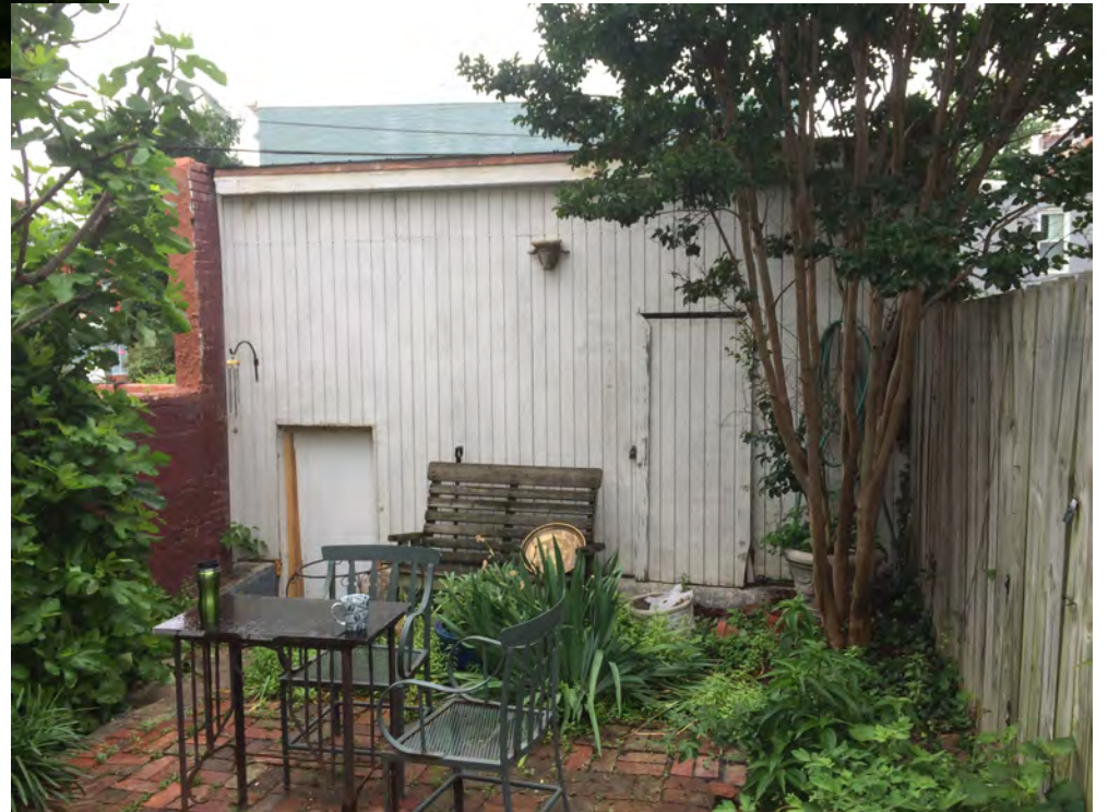
VIEW FROM YARD, EXISTING GARAGE
