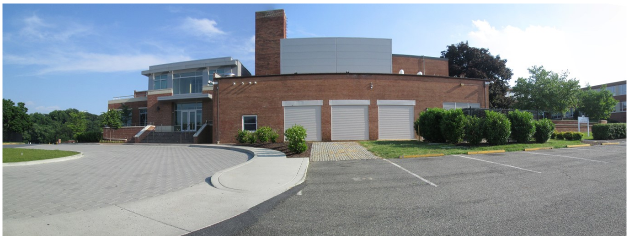
View of boiler room, facing south
