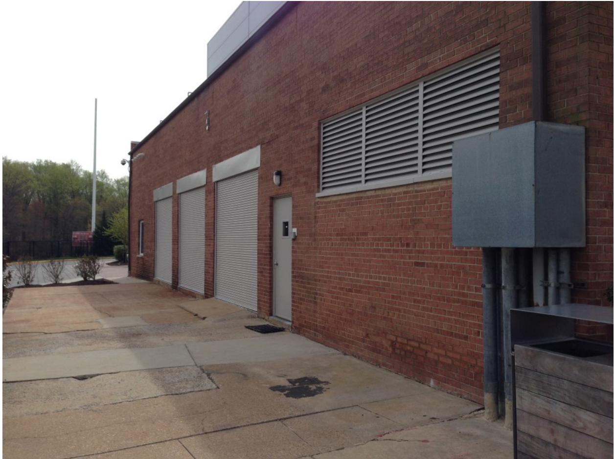
View of the boiler room, facing southeast
