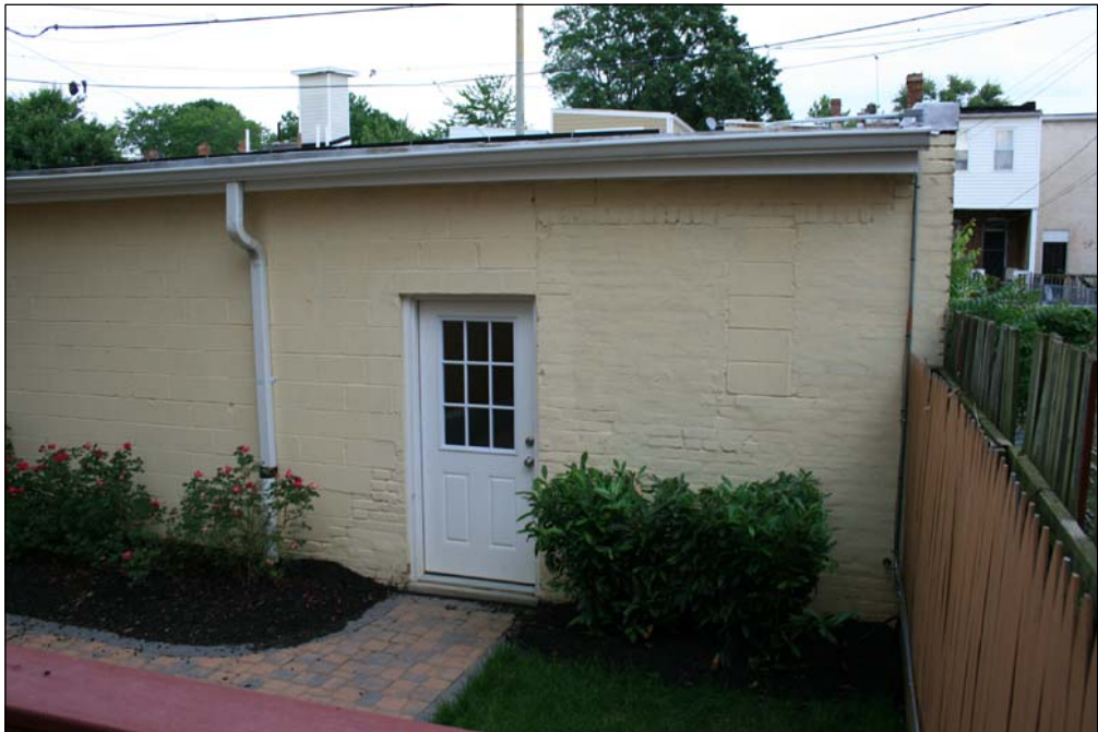
View from rear yard towards alley
