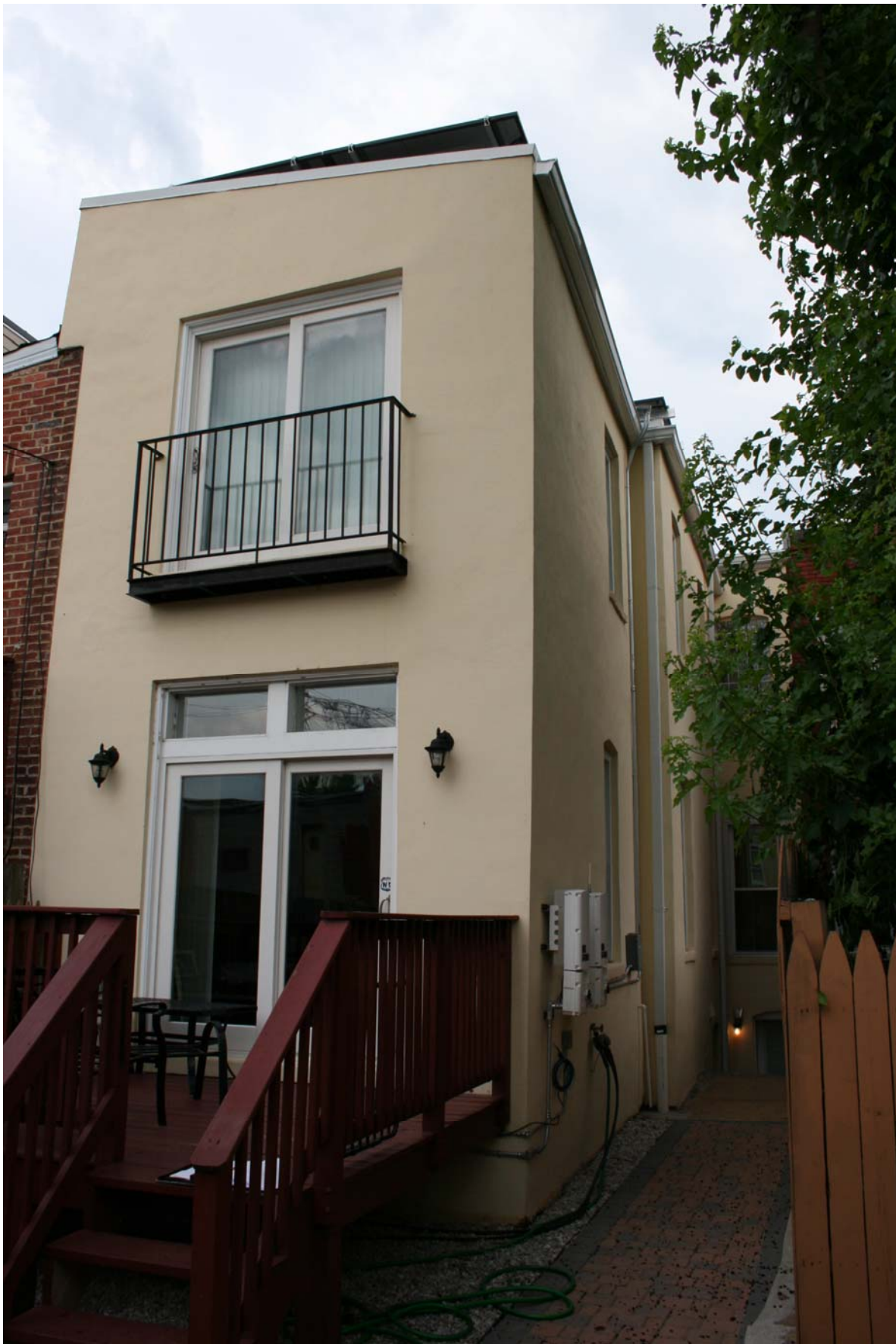
View of 815 8 th Street NE from rear yard
