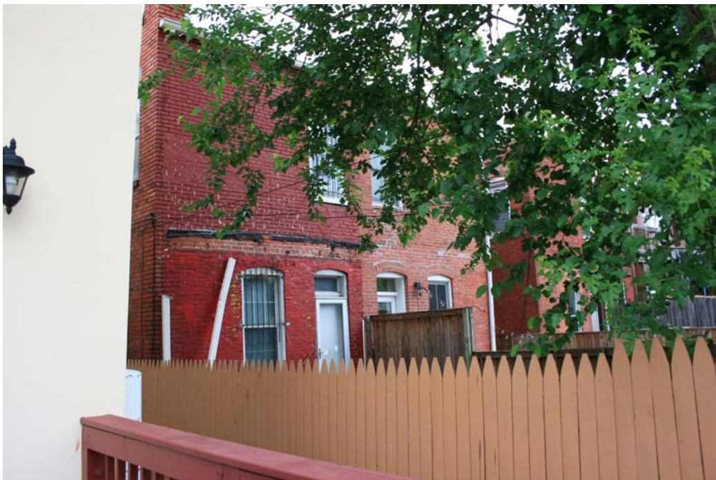
View from rear yard towards 817 8 th Street NE
