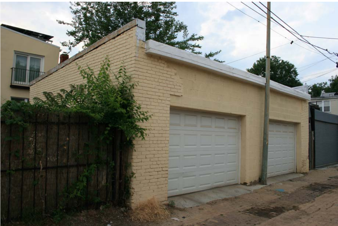
View of existing garage from alley
