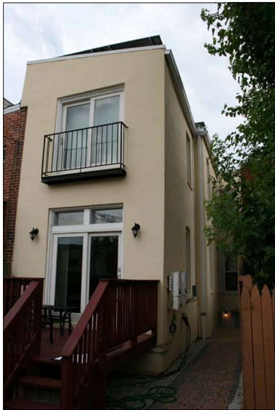
View from rear yard
