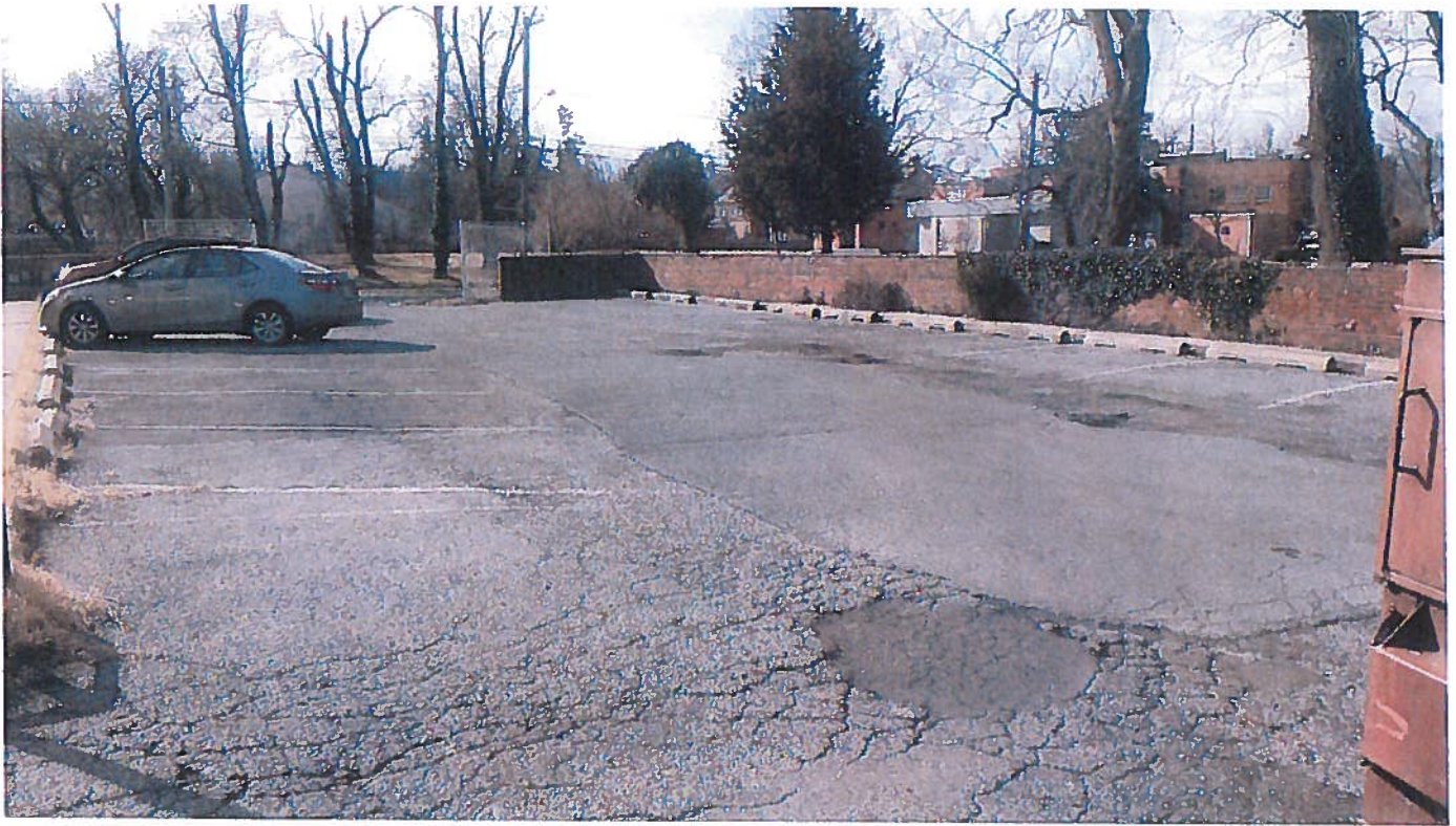
View from Rear of Parking Lot (Facing Tuckerman Street NW)
