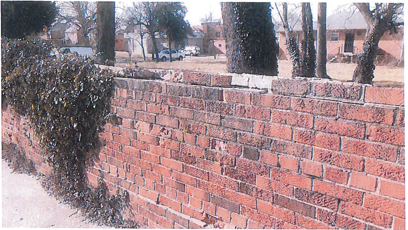
Brick Wall on the Western Boundary of the Parking Lot
