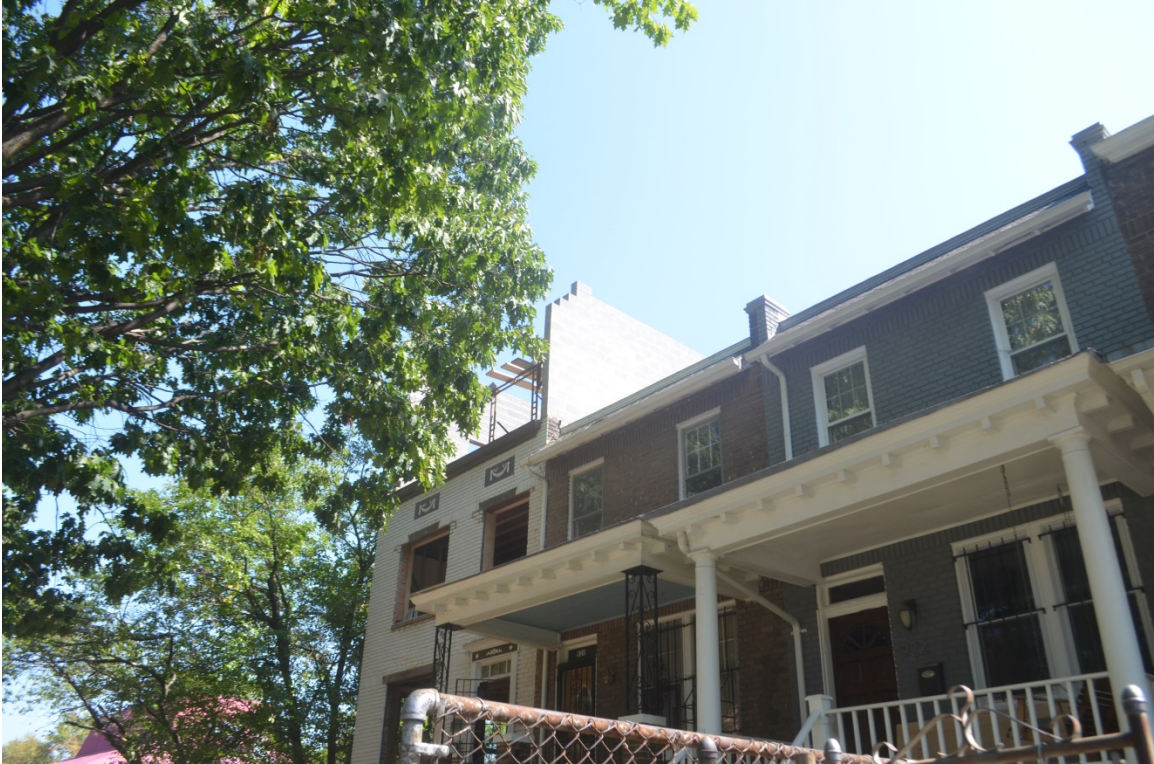
Figure 3 – 918 14 th Street, SE – 3-story addition in progress (north of applicant property)
