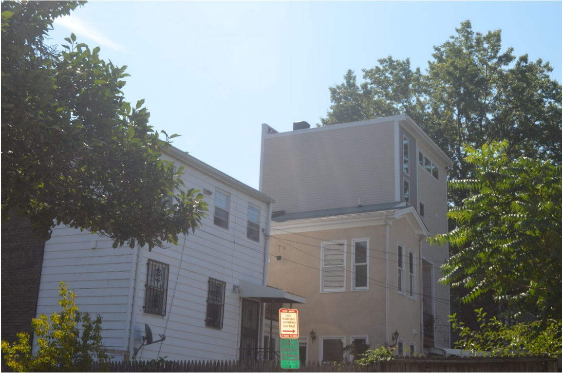
Figure 4 – 951 14 th Street, SE – 3-story addition off back of property (west of applicant property)
