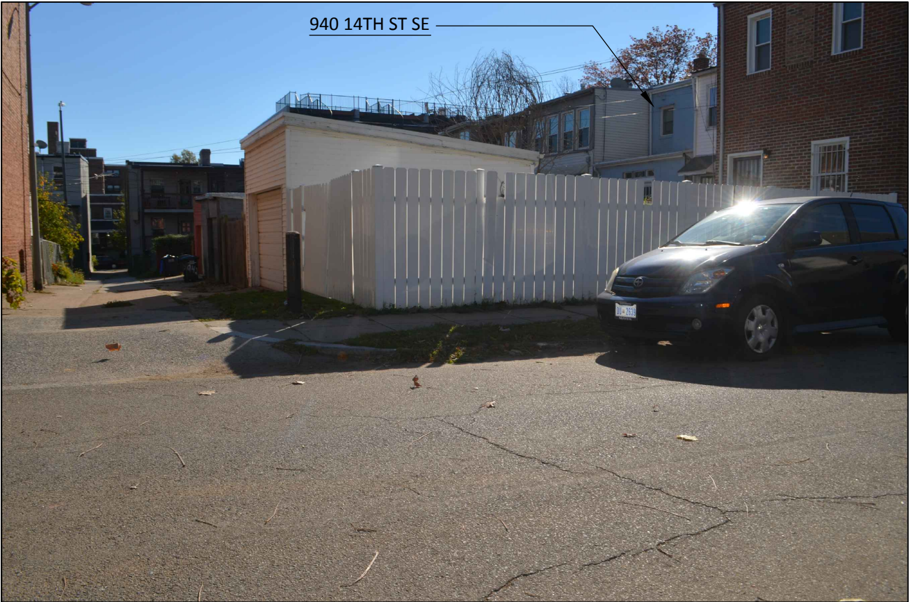
#4: VIEW OF REAR ALLEY FROM IVES PLACE SE LOOKING SOUTHWEST
