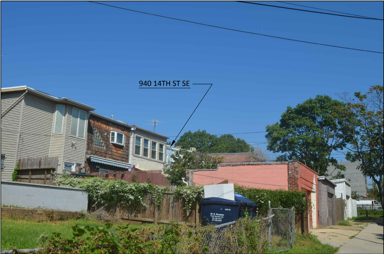
#3: VIEW OF REAR ALLEY LOOKING NORTHWEST
