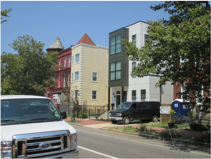
EXISTING VIEW LOOKING WEST
