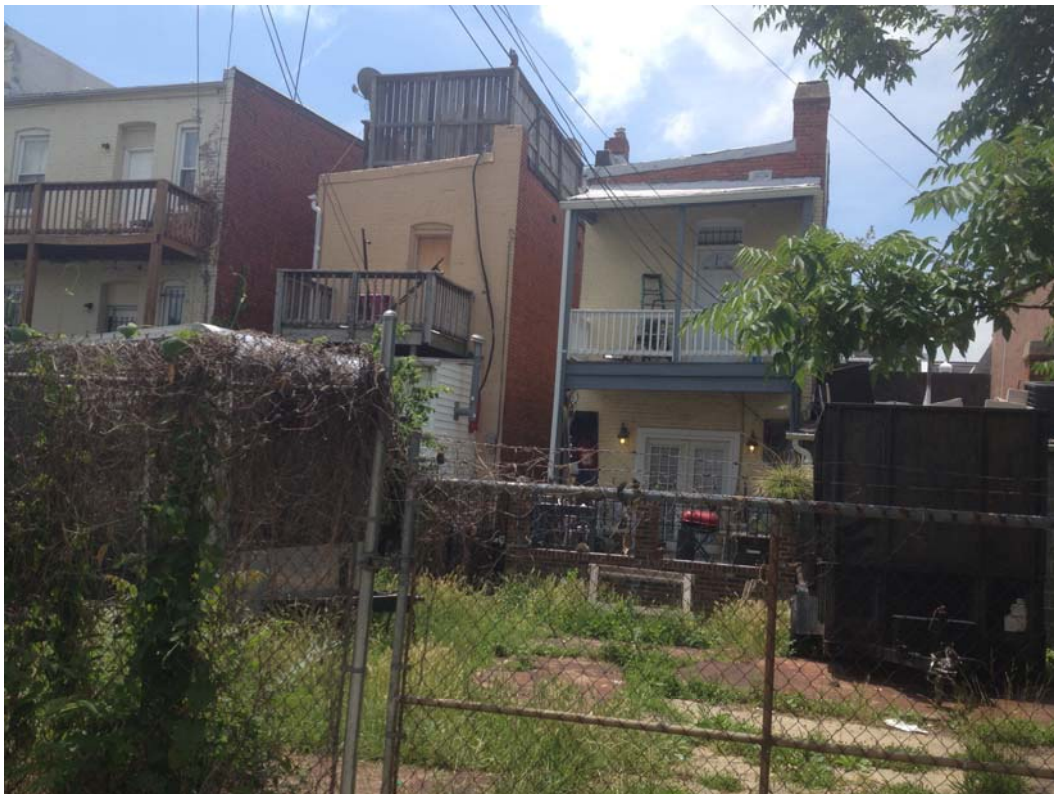
View from Rear Alley (existing structure behind trailer)
